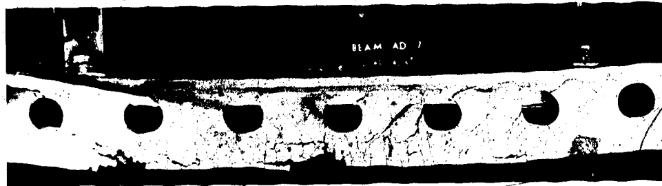
PLATE 4. BEAM AD-7 CRACKING AND FAILURE PATTERNS
