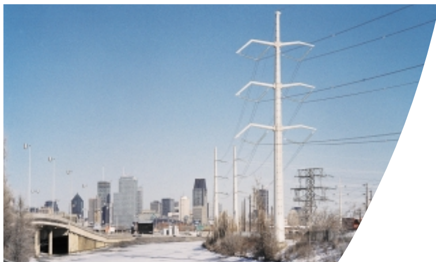
Aqueduc - Atwater - Viger 315-kV line
