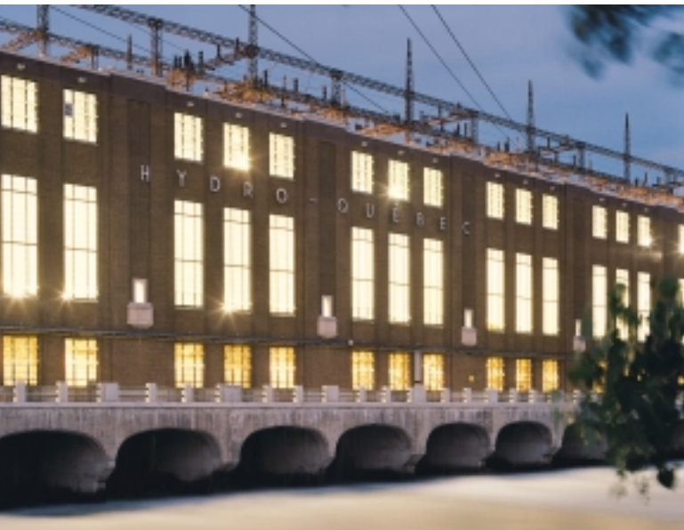
Beauharnois generating station
