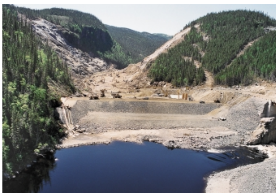
Sainte-Marguerite-3 construction site
