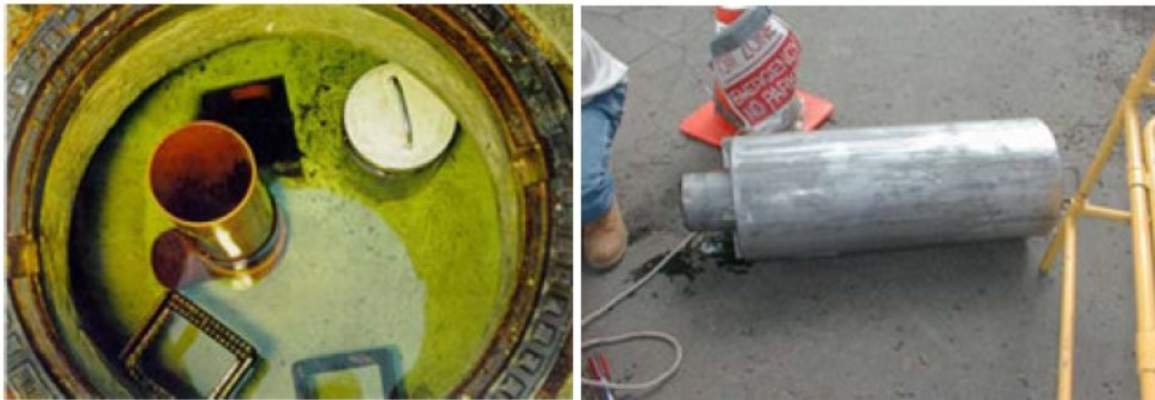
Figure 2-6. Flushing devices (Dettmar et al. , 2002; Fan, 2004)
