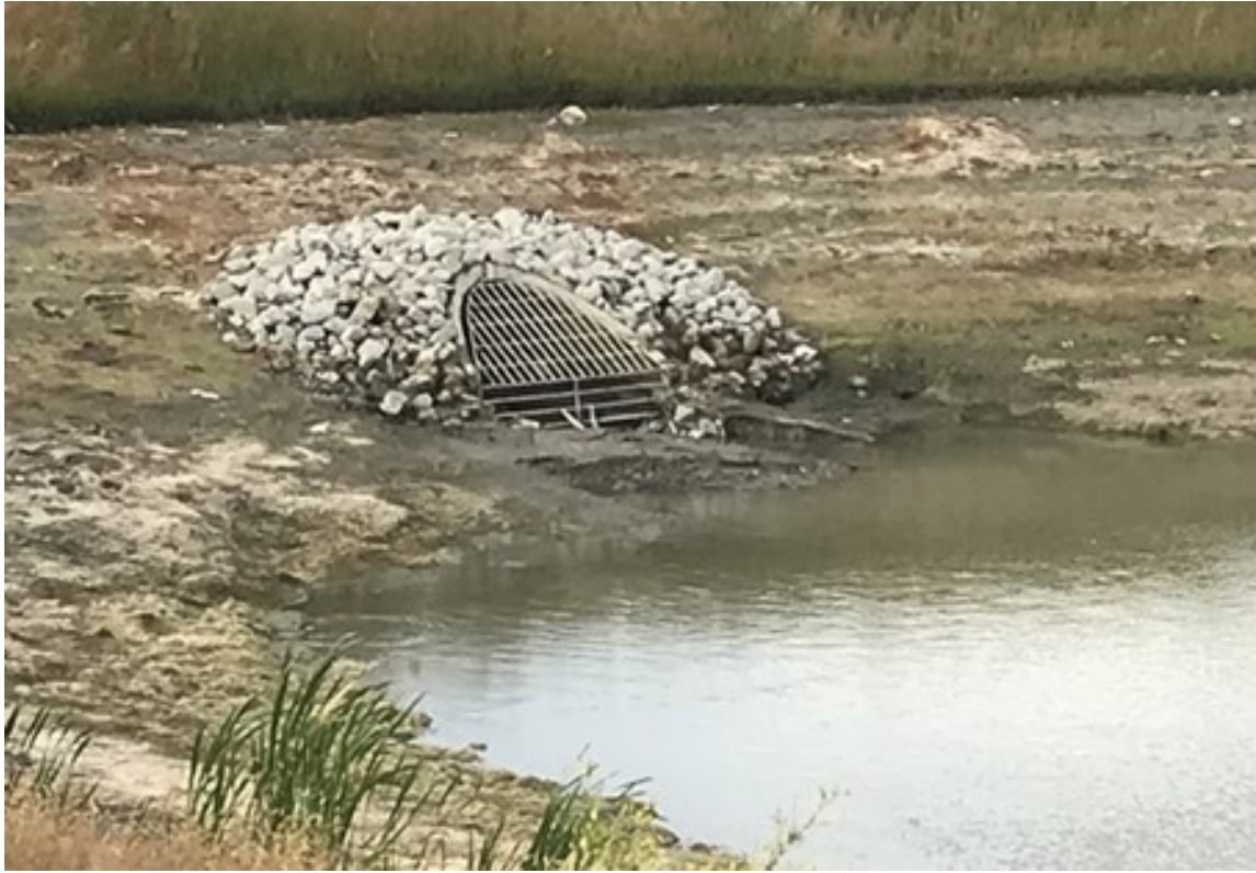
Figure 1-2. Submerged storm sewer outlet (going to a drained storm water pond)
