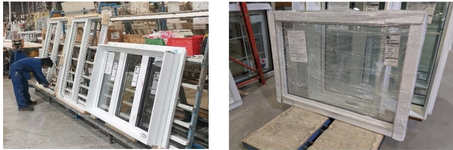
Figure 17 Glazing and wrapping.
