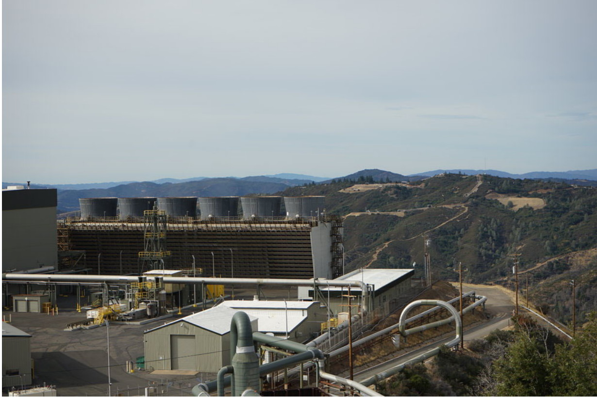
Figure A.36. One of the many power plants at the Geysers geothermal field, the world's largest geothermal power producer. In the background, numerous steam pipes from various wells are visible.
