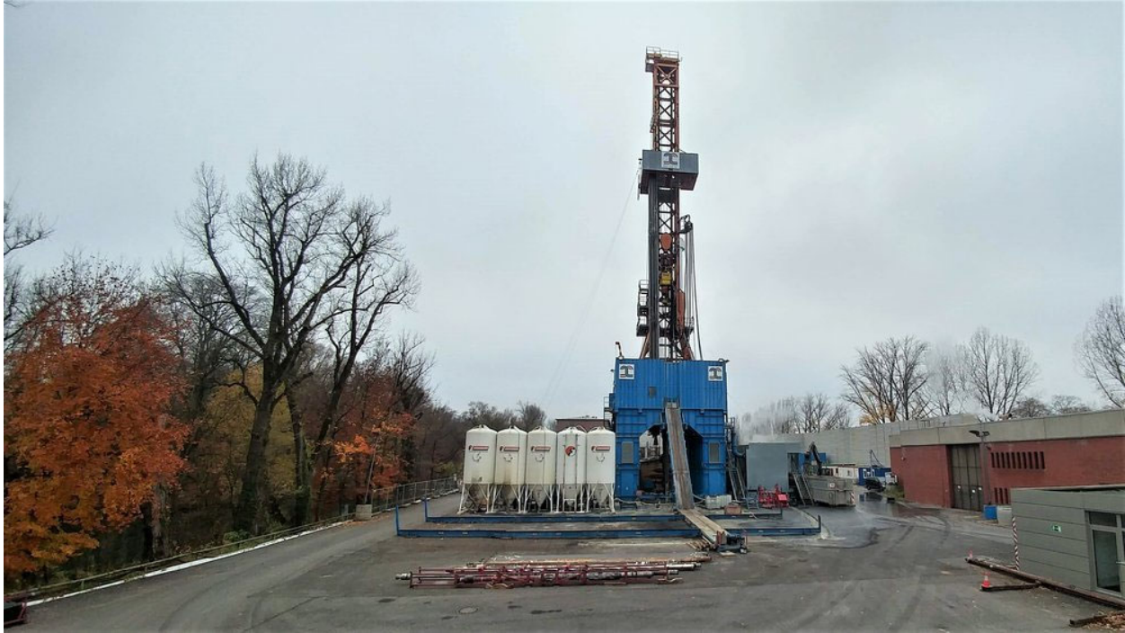
Figure A.41. The Schaftlarnstrasse geothermal drilling operation near the Munich city center. Electronics had to be turned off while on the drill rig, so this is the best photo I've got!
