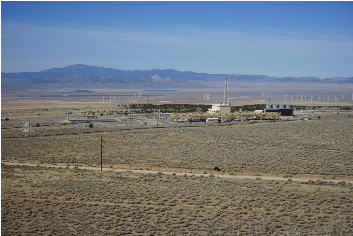
Figure A.34. The Milford Renewable Energy Corridor, looking WNW. In the foreground, the Blundell Geothermal Power Plant produces 34 MW of power from a hydrothermal system that appears to be bounded by a steep fault that roughly corresponds to the treed hillside behind the plant. The Milford FORGE site will be between the rows of wind turbines on the right side of the image. Across the valley, a large solar farm also produces electricity.
