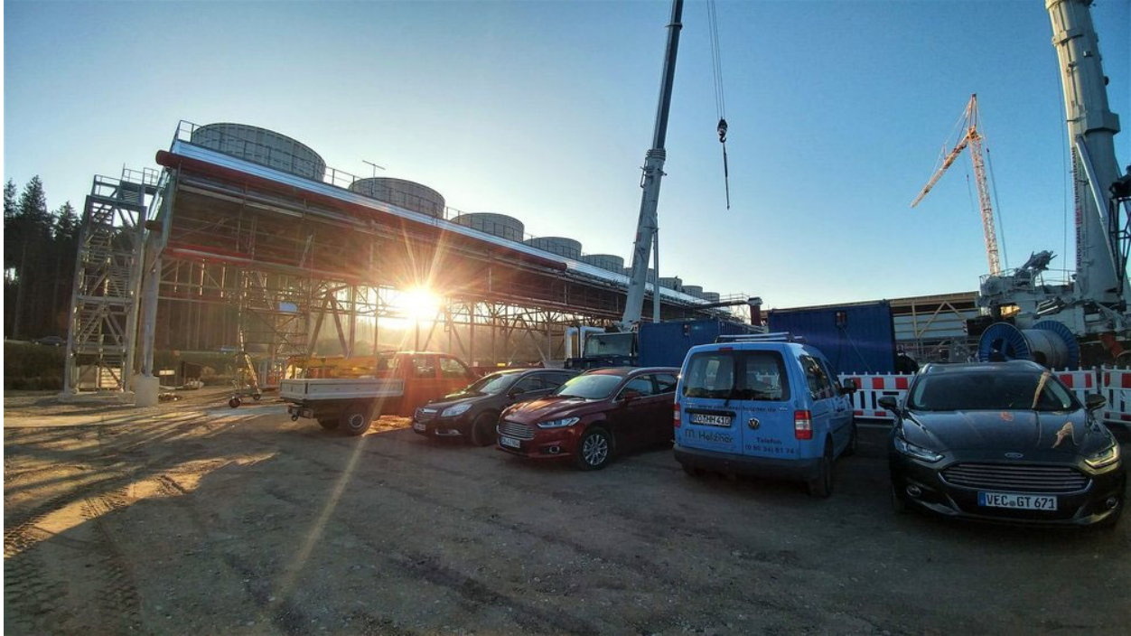
Figure A.42. Cooling towers at Holzkirchen. Working fluid must be cooled to create a pressure differential to drive the turbines.
