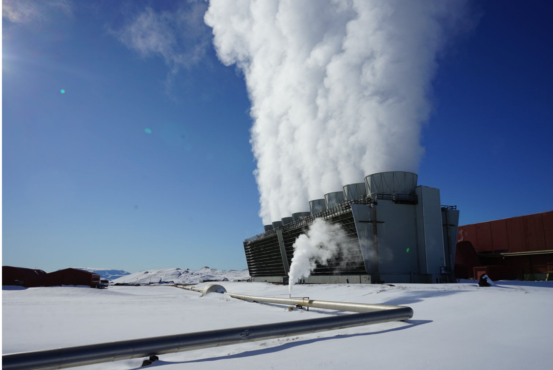
Figure A.20. Cooling towers at the Krafla Power Plant
