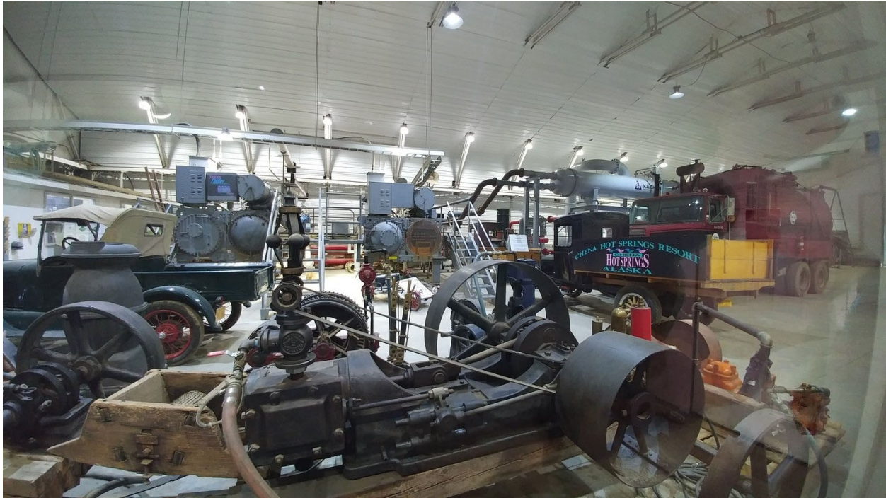
Figure A.8. The power plant at Chena Hot Springs along with an assortment of older machinery. Three Organic Rankine Cycle (ORC) engines are installed, producing approx. 400kWh.
