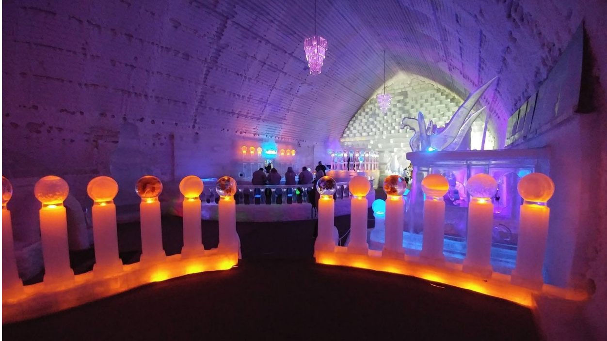
Figure A.11. The Ice Museum at Chena Hot Springs, kept cold year-round with a geothermally powered absorption chiller.
