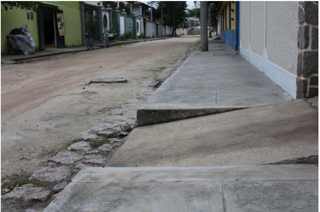
Figure 9. Ramps on the sidewalks
