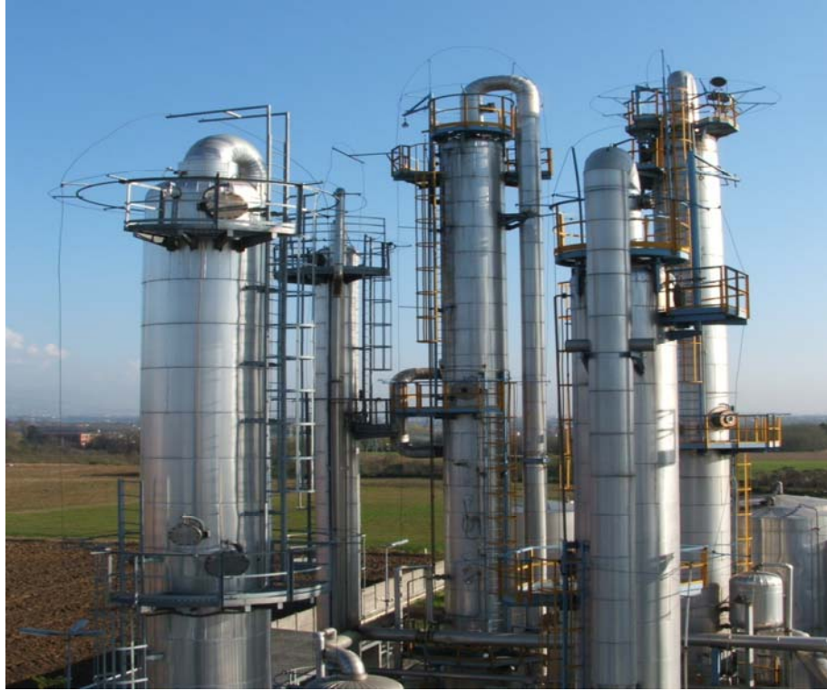
Figure 1-4 A typical distillation tower in industry
