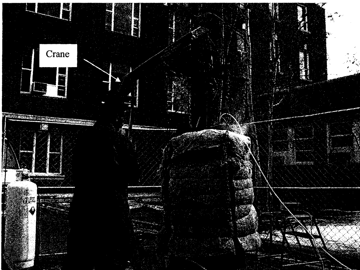
Figure 3-6 Apparatus hanging from crane
