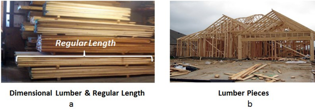
Figure 3.7: Examples of dimensional lumber, regular length, and lumber pieces (Pekin Hardwood 2015; Build Your Own House 2011).
