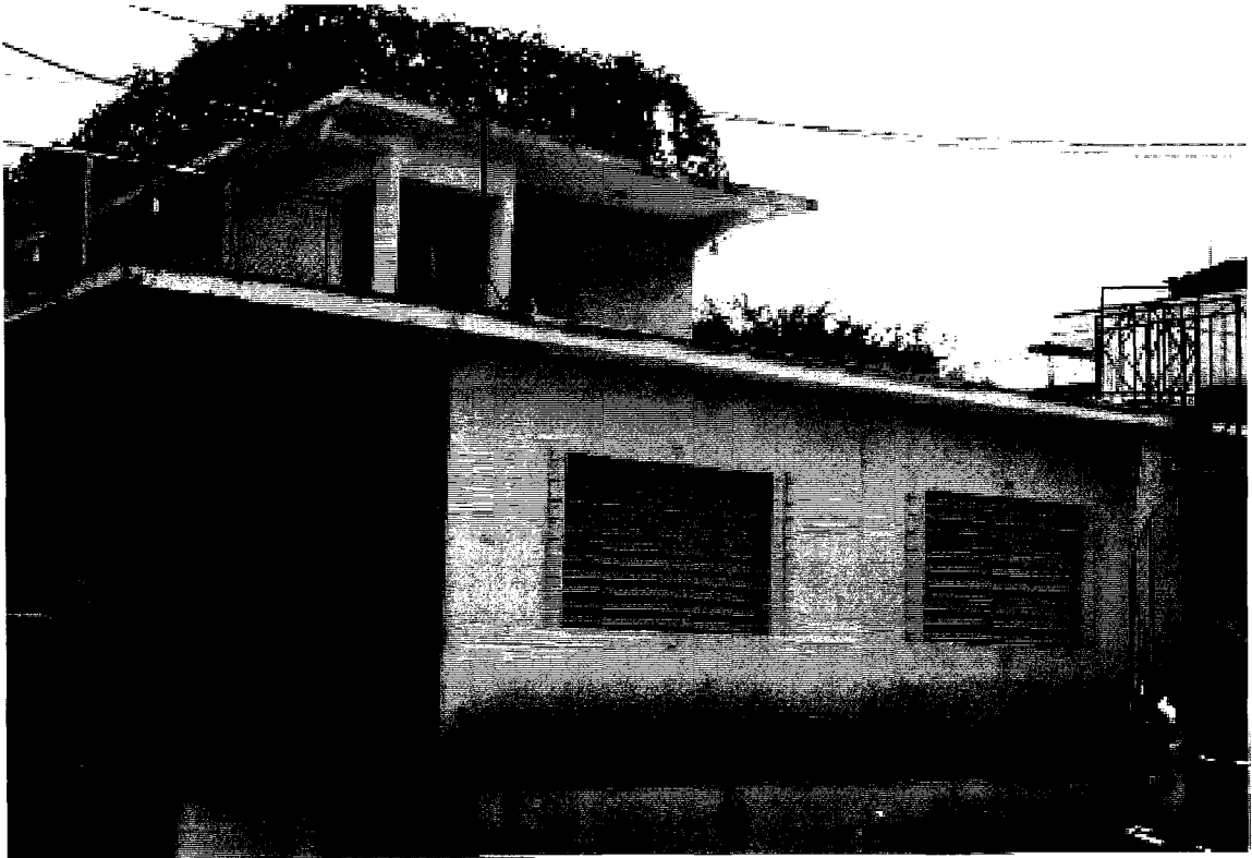
Figure 9: A typical post-Revolutionary Cuban home similar to that in which the researcher lived during her field studies. Construction is of cinder block and concrete.
