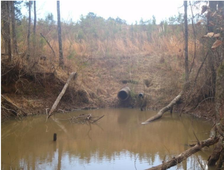
Figure A-6 the tunnel on the south side with the towards the drainage zone.
