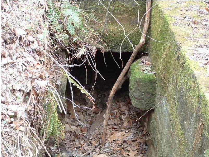
Figure A-9 This is the south side entrance into tunnel 4, this tunnel is created of concrete blocks and is approximately 0.5m.x0.75m.
