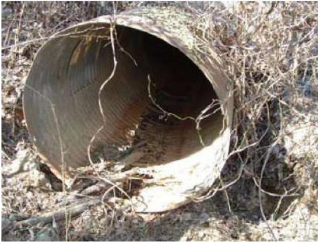
Figure A-3 This is the south entrance of the tunnel
