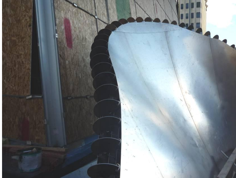
Figure 8 Prefabricated Borealis panel prior to installation on building.
