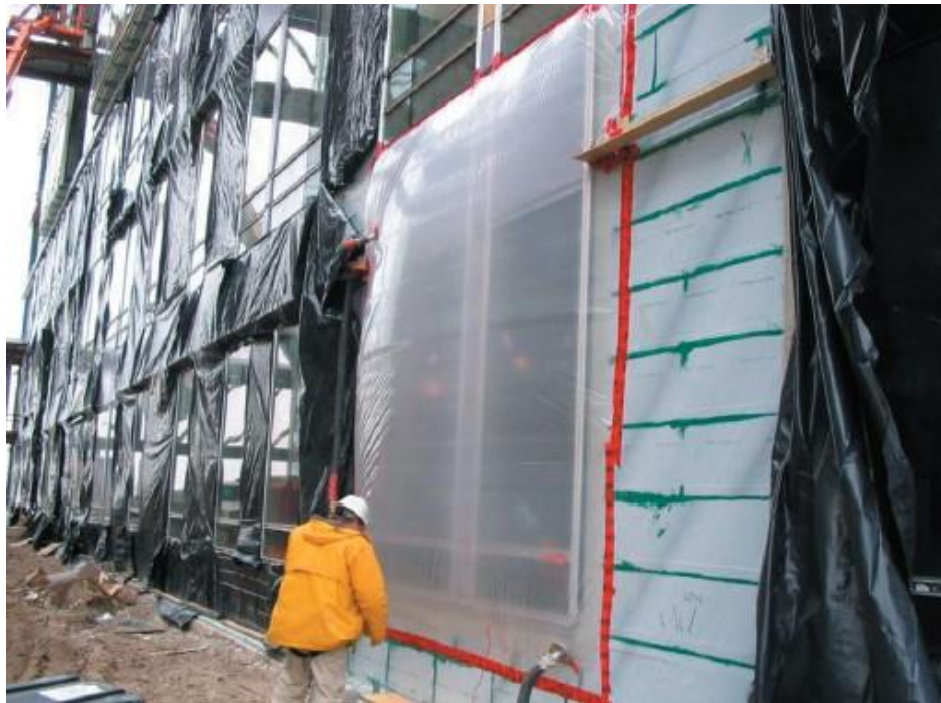
Figure 7—Airtightness test conducted by ASTM E 1186 (Knight and Boyle, 2010)
