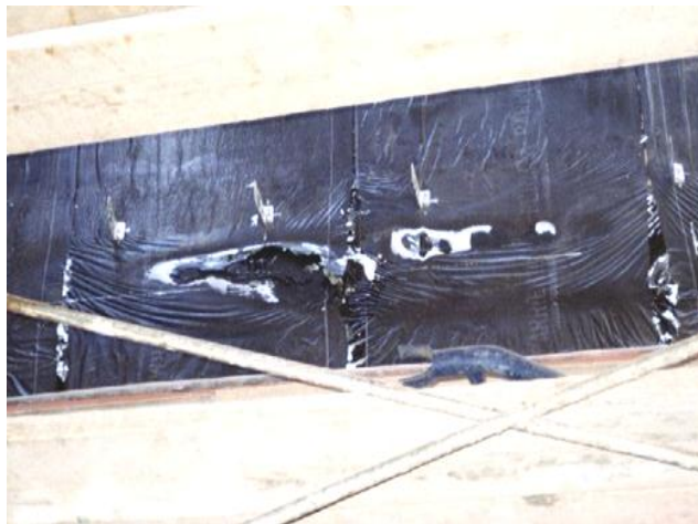
Figure 26 - Melted membrane caused by the fire during initial construction
