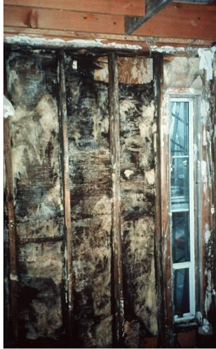
Figure 20- Mouldy insulation in a wood stud wall caused by water entering the wall cavity (photo courtesy of Read Jones Christoffersen)
