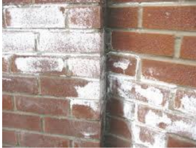
Figure 17 – Efflorescence staining on a building’s brick façade indicates moisture issues within the wall cavity (photo courtesy of Read Jones Christoffersen)
