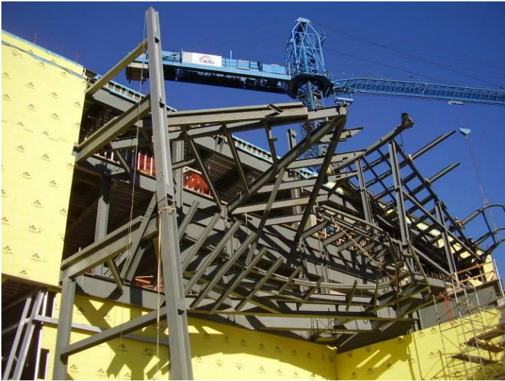
Figure 10: Structural steel framing for Borealis.
