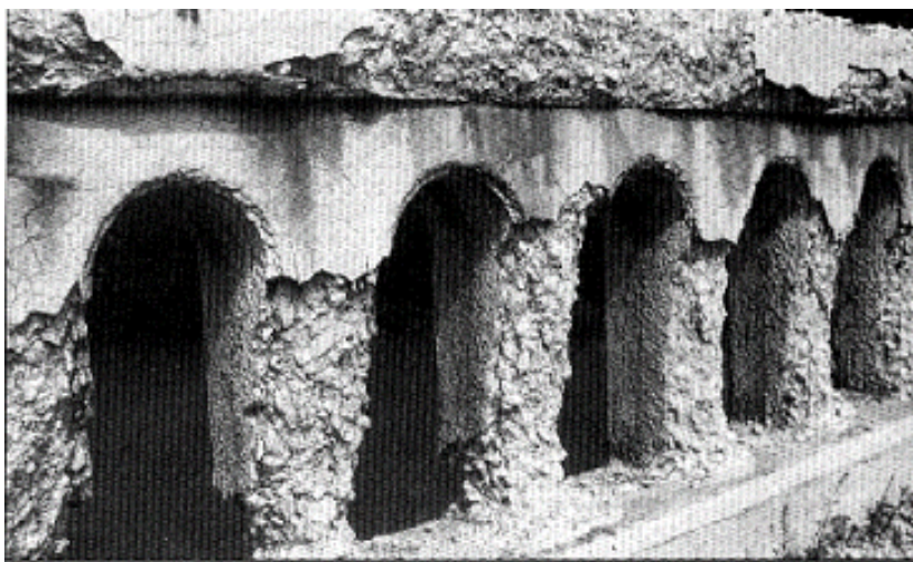
Figure 18 – The effects of freeze-thaw on an older structure (Portland Cement Association, 1998)
