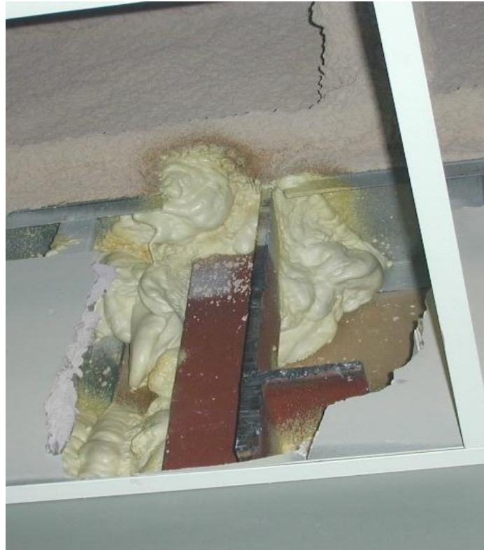
Figure 23 - Wall penetration repair had been completed after building envelope failure was first expected in hopes of solving the building envelope issues
