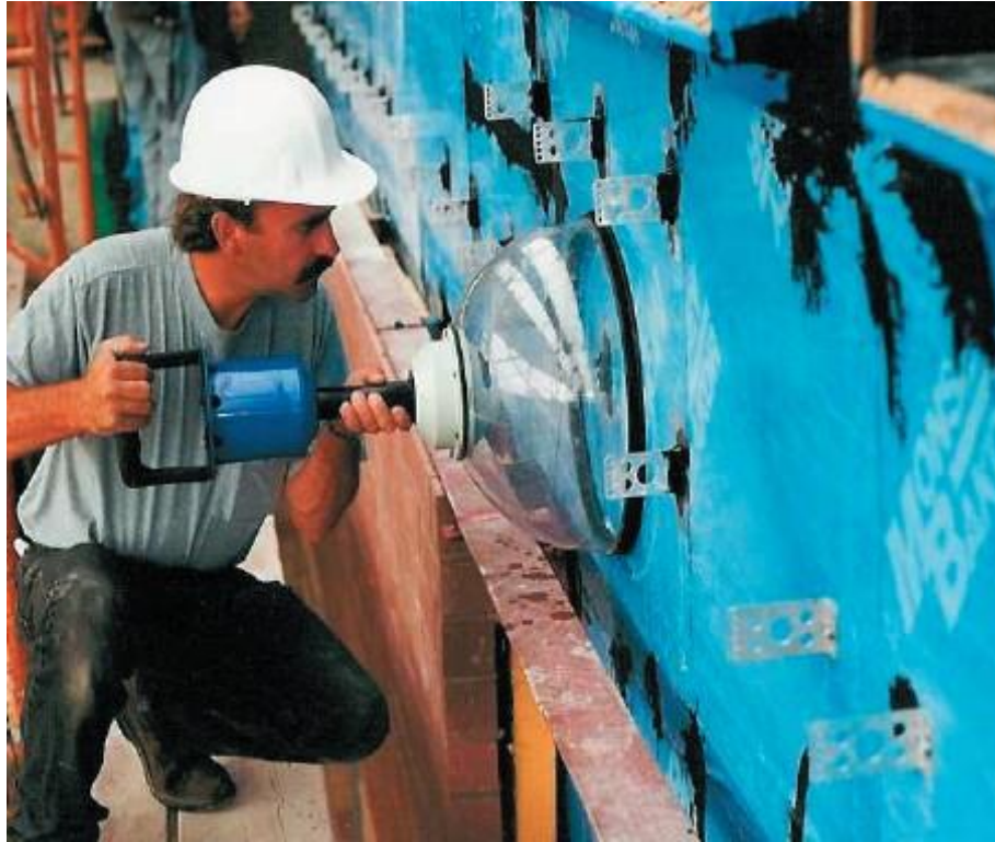
Figure 8—Airtightness test conducted per ASTM E 1186(Knight and Boyle, 2010)
