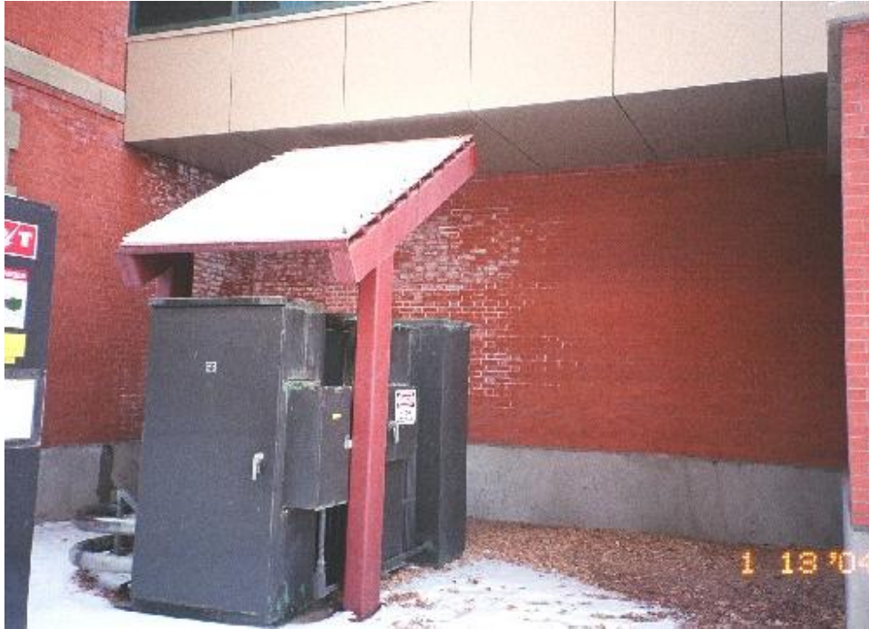
Figure 24 - Efflorescence stained brick façade on the exterior of Building X. This indicated condensation issues occurring behind the façade
