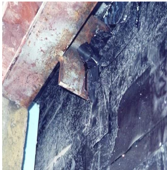
Figure 25 - Knife edge support at brick angle location where heat loss was present. Membrane appeared to be haphazardly applied
