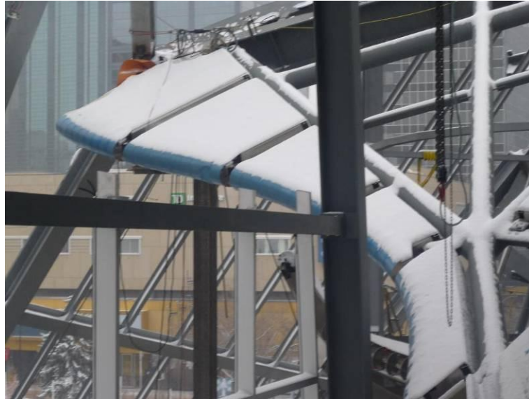
Figure 6: Snow accumulation on Borealis during construction.
