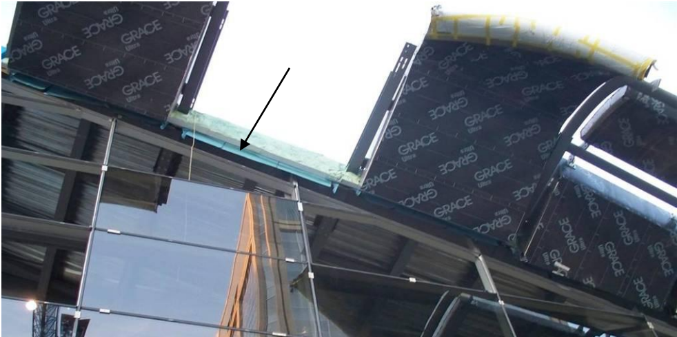
Figure 12: Foam applied to exterior steel prior to panel erection.
