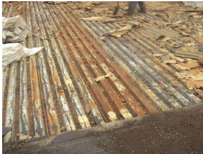
Figure 16 - Corrosion of a metal roof deck caused by water ingress. If left unrepaired, corrosion can cause structural failure in structural metal components such as the roof deck (O'Reilly, 2006)
