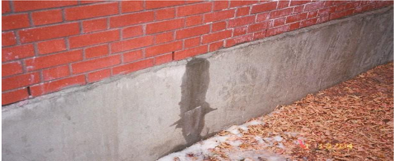
Figure 19 – Horizontal shrinkage cracks of a concrete foundation wall allow for water to seep through the crack (photo courtesy of Read Jones Christoffersen)
