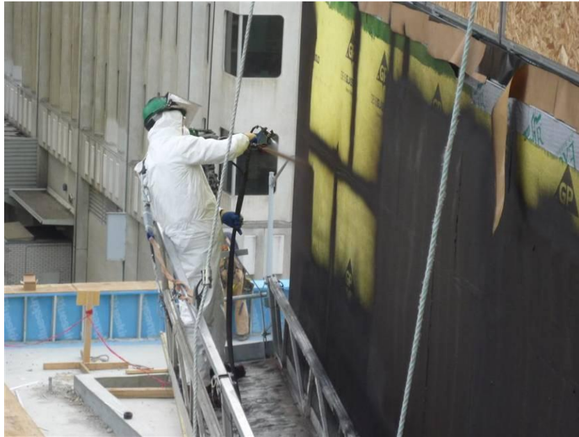
Figure 13: Application of sprayed membrane.
