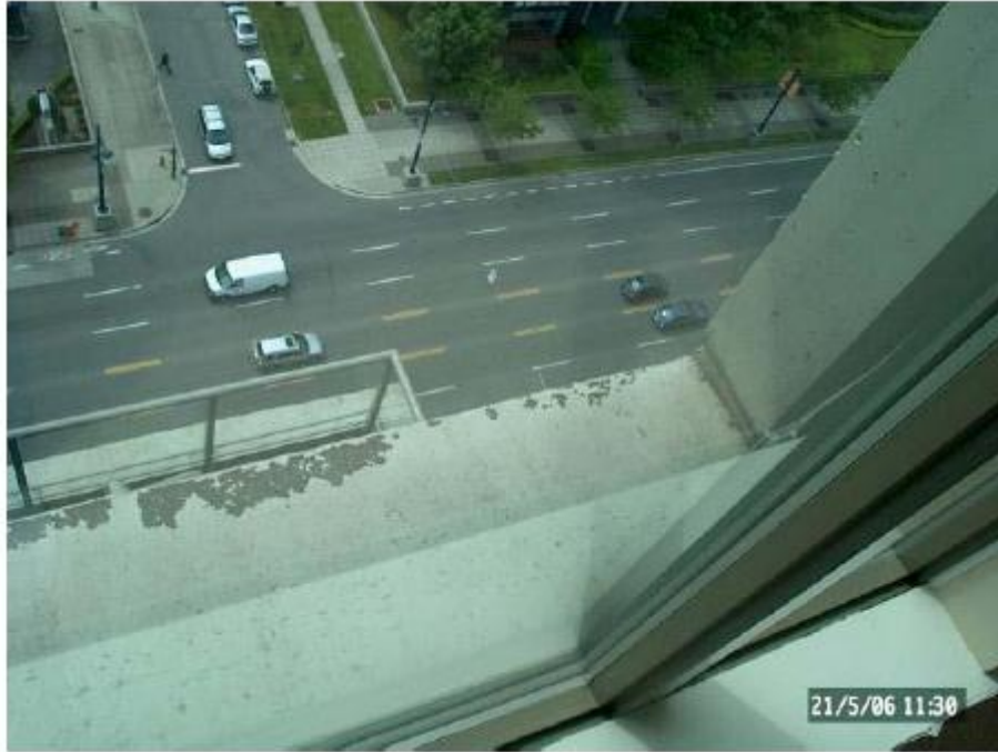
Figure 15 - Slab Projection past Glazing System showing loss of coating from the concrete (Busque, 2010)
