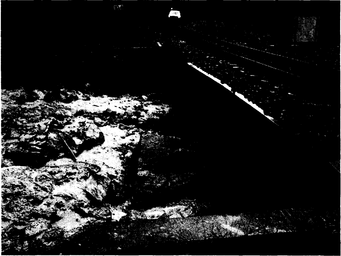
Figure 4.9. Debris flow deposition within channel 'd' in basin 54.0 on July 18, 2001. Similar deposition channel 'a' in basin 53.6 caused track failure (Chapter 2). Photo courtesy Tim Keegan.
