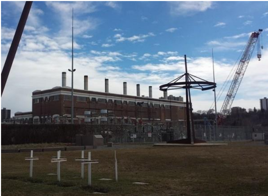
Fig. 15. Memorial and EPCOR power plant (Glang)
