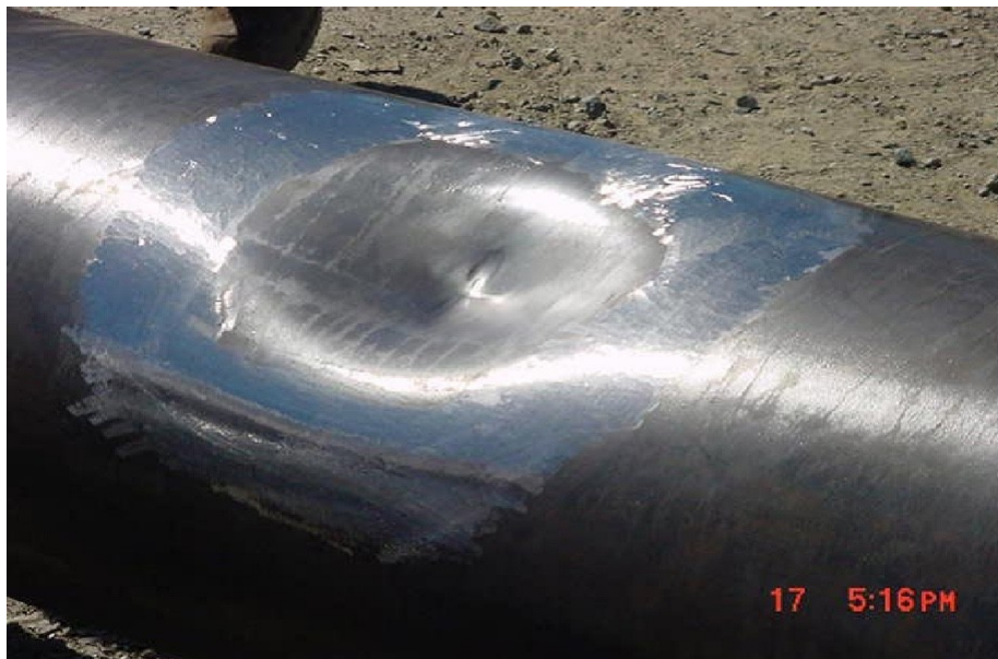
Figure 12: Photograph of a dent in the pipeline [36].
