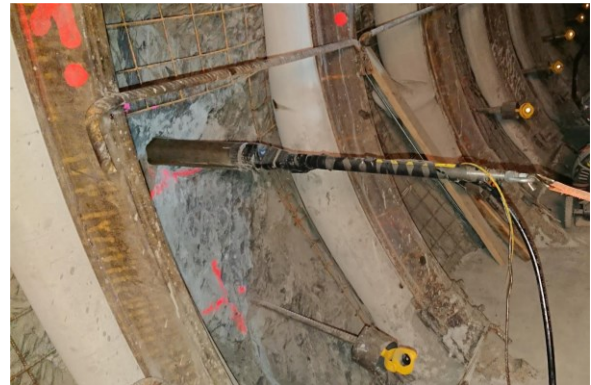
Figure A- 12. Deployment of pressuremeter in borehole BGC-A6 (horizontal)
