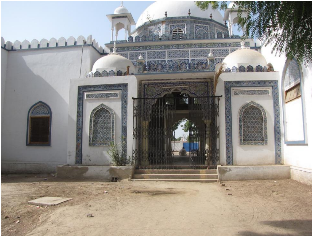
Figure 16: Outer facade of the Shah jo Raag School, 2009
