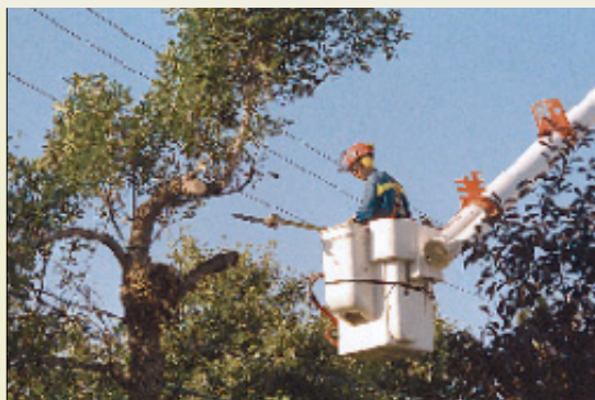
All vegetation control on the distribution system is done mechanically.
