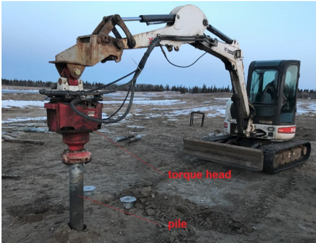
Figure 3.4. Pile installation equipment at Sandpit.
