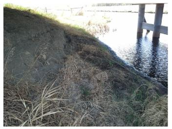
Photo No.: Photos-20180516-175804.jpg Description: Erosion potential
