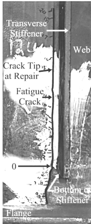
Figure 4-17 Fatigue Crack on West Face of Joint 12, Specimen 3
