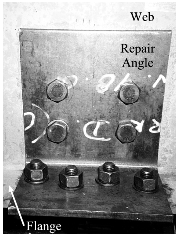
Figure 3-8 Typical Repair Angle Connected to Web and Bottom Flange
