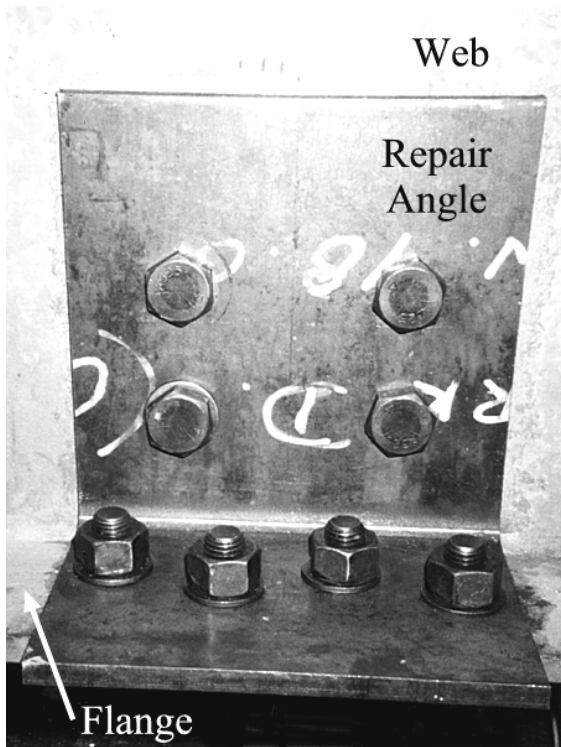
Figure 4-27 Repair Angle at Joint 11, Specimen 4
