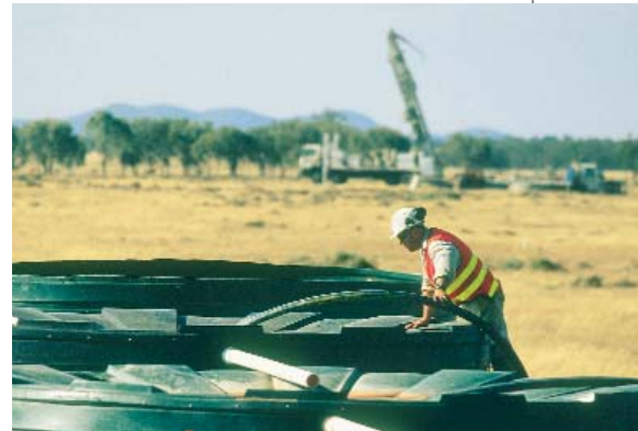
Serge Smolonogov, exploration driller, checks drilling water holding tanks at Cowal, New South Wales. Removable holding tanks eliminate the requirement for excavated sumps at this drill site.
