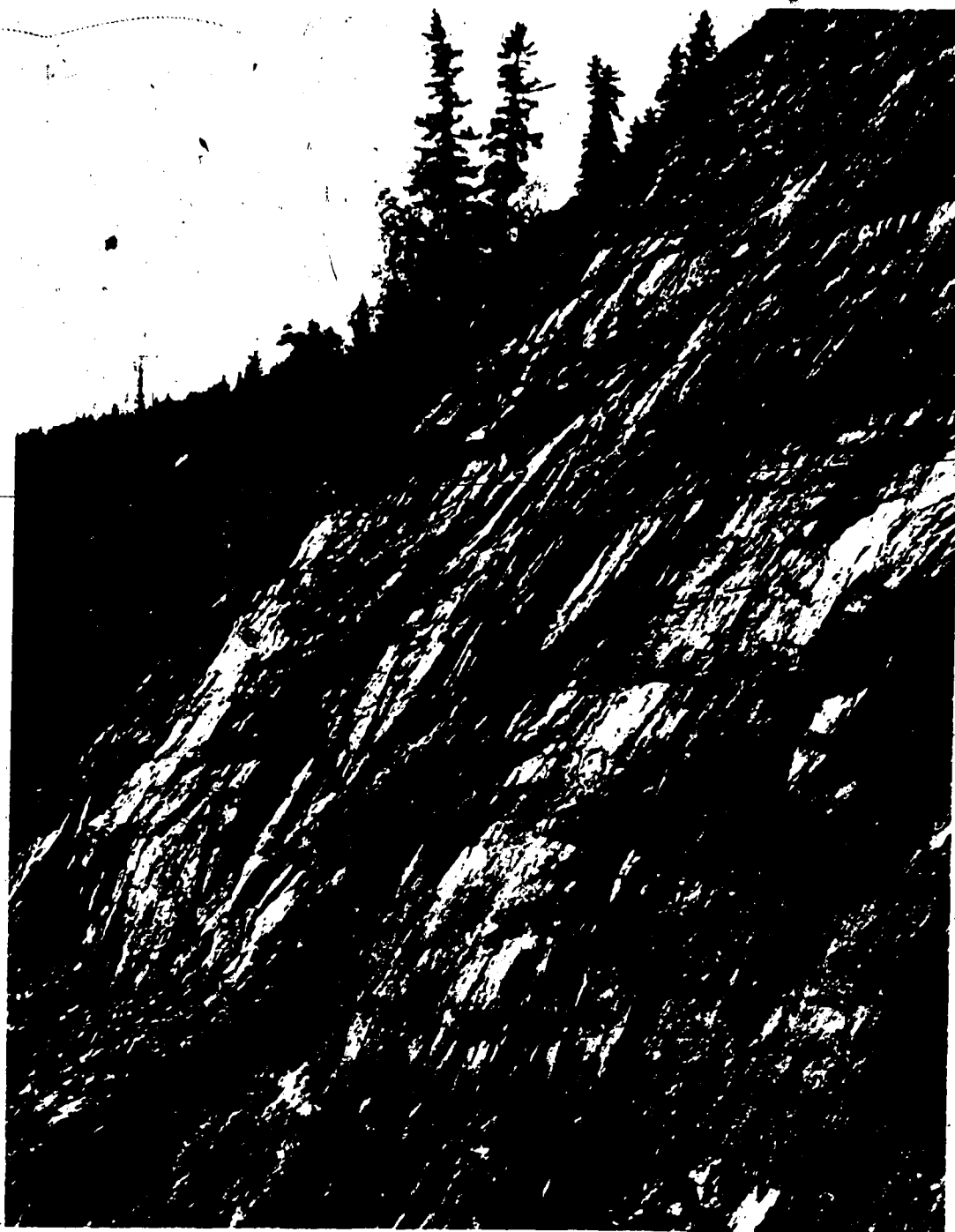
PLATE 3.4 Well-developed Exfoliation Fractures. Slope #16a. Slope angle is about 65° over a 20m height.
