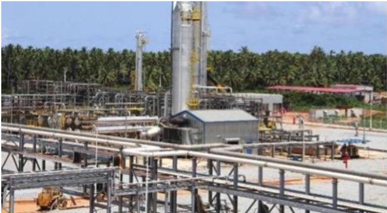
Figure 2: Atuabo Gas Plant (a portion of plant under construction)
