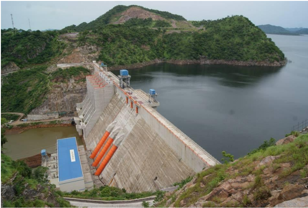
Figure 5: Bui Hydro Dam
