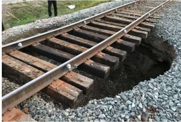
Figure 3.6: Sinkhole Underlying Track 1
