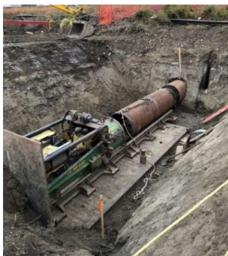
Figure 2.1: Horizontal Auger Boring Construction [4]
