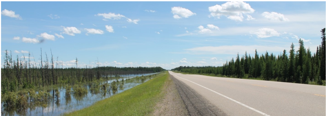
Figure 1-1: Photograph depicting a road-fragmented peatland with flooding on the left side of the road (water source; up flow-side) and increased tree growth and recruitment on the right side (down flow-side). This location is near Conklin, Alberta on Hwy 881 ( 55^{\circ}15'01.6''N 111^{\circ}19'17.4''W , facing south, May 2016, photo by Caitlin Willier).
