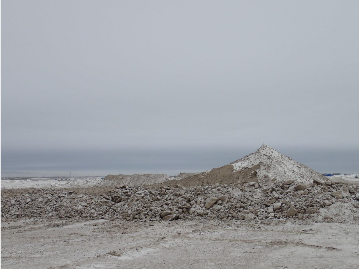
Winter Photo (c), Table 8. Steep slopes produced when pushing frozen soil and snow.
