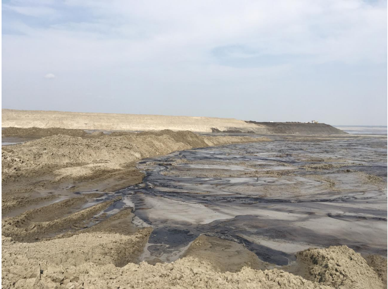
Summer Photo (d), Table 7. View of tailings discharge are with tailings berm (~20 m high) in background.
