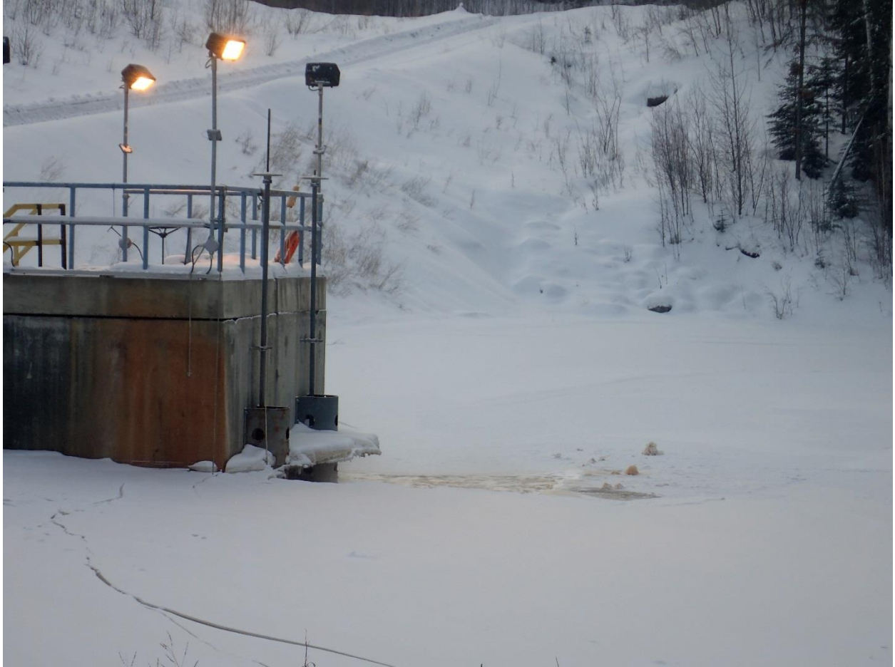
Winter Photo (i), Table 8. Pump station downslope of tailings pond dam; open water can be seen at pond intake.
