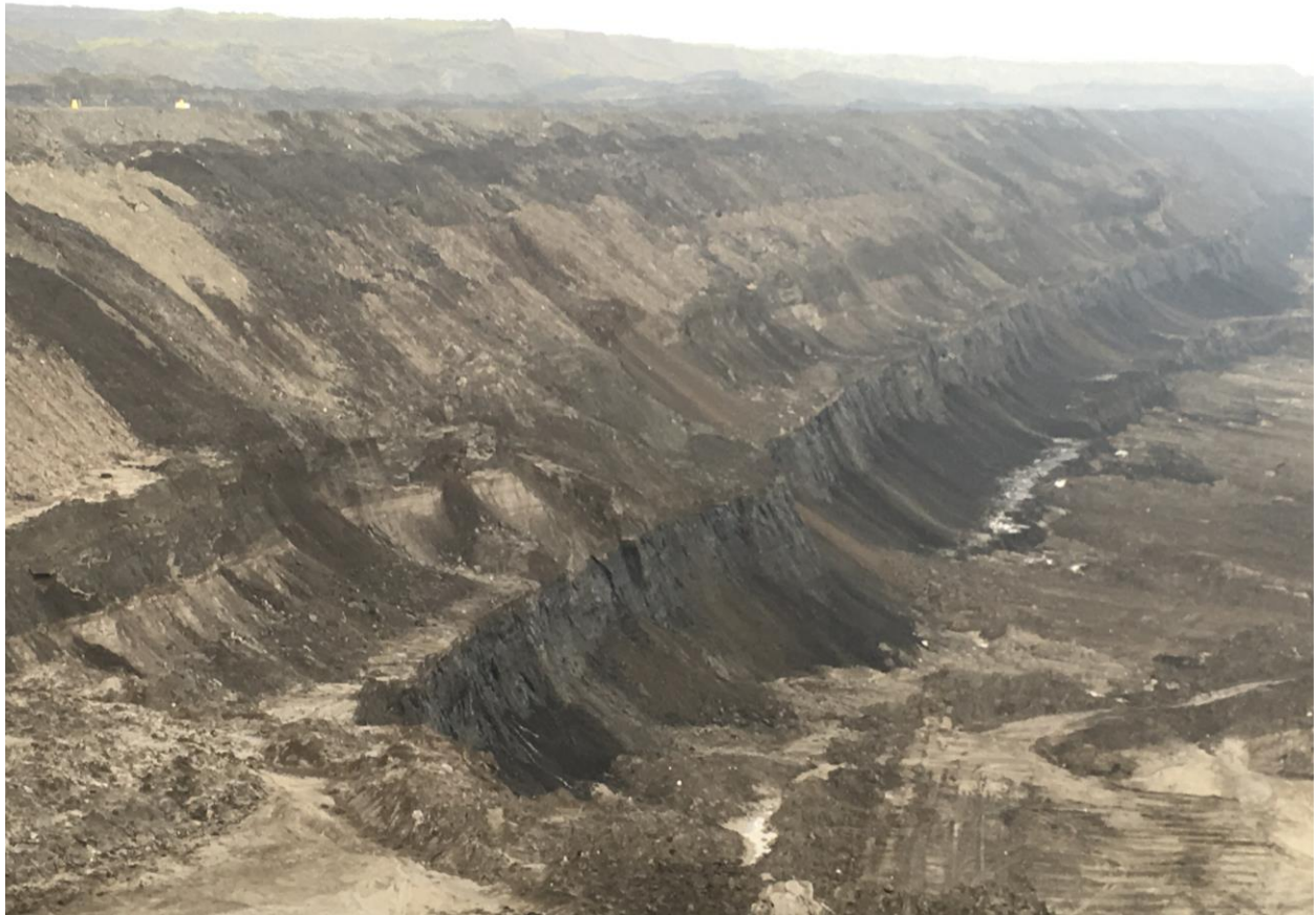
Summer Photo (a), Table 7. View of the open pit (~30 m deep). Steep slopes typical of mining operations. A failed slope can be seen (top) at an inactive pit area.
