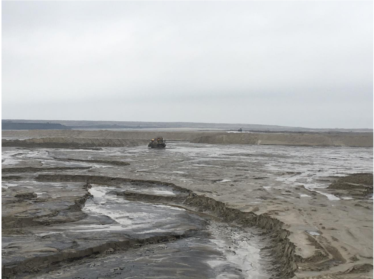
Summer Photo (e), Table 7. Bulldozer at work in soft ground at tailings discharge area.
