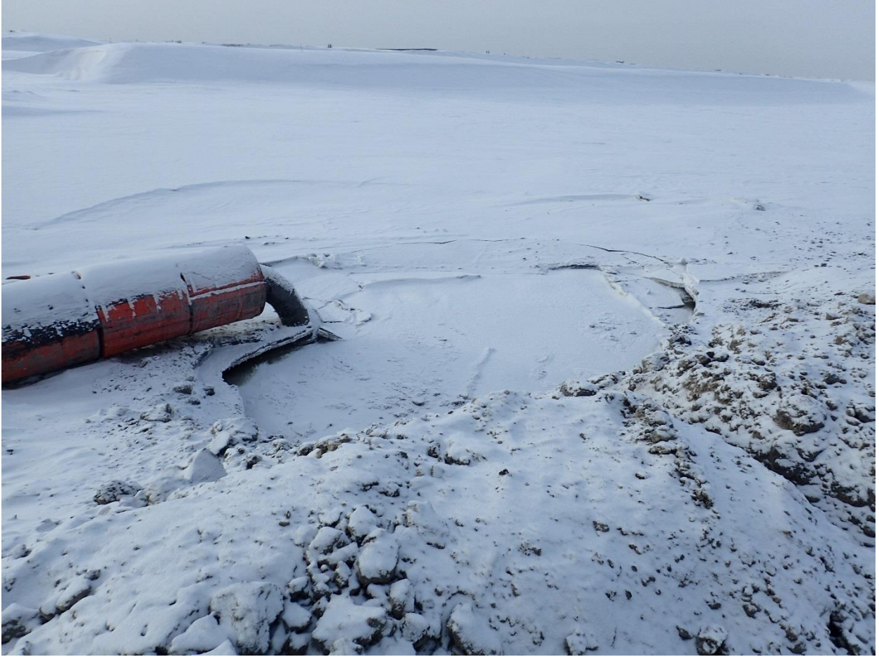
Winter Photo (j), Table 8. Frozen sump pump station
