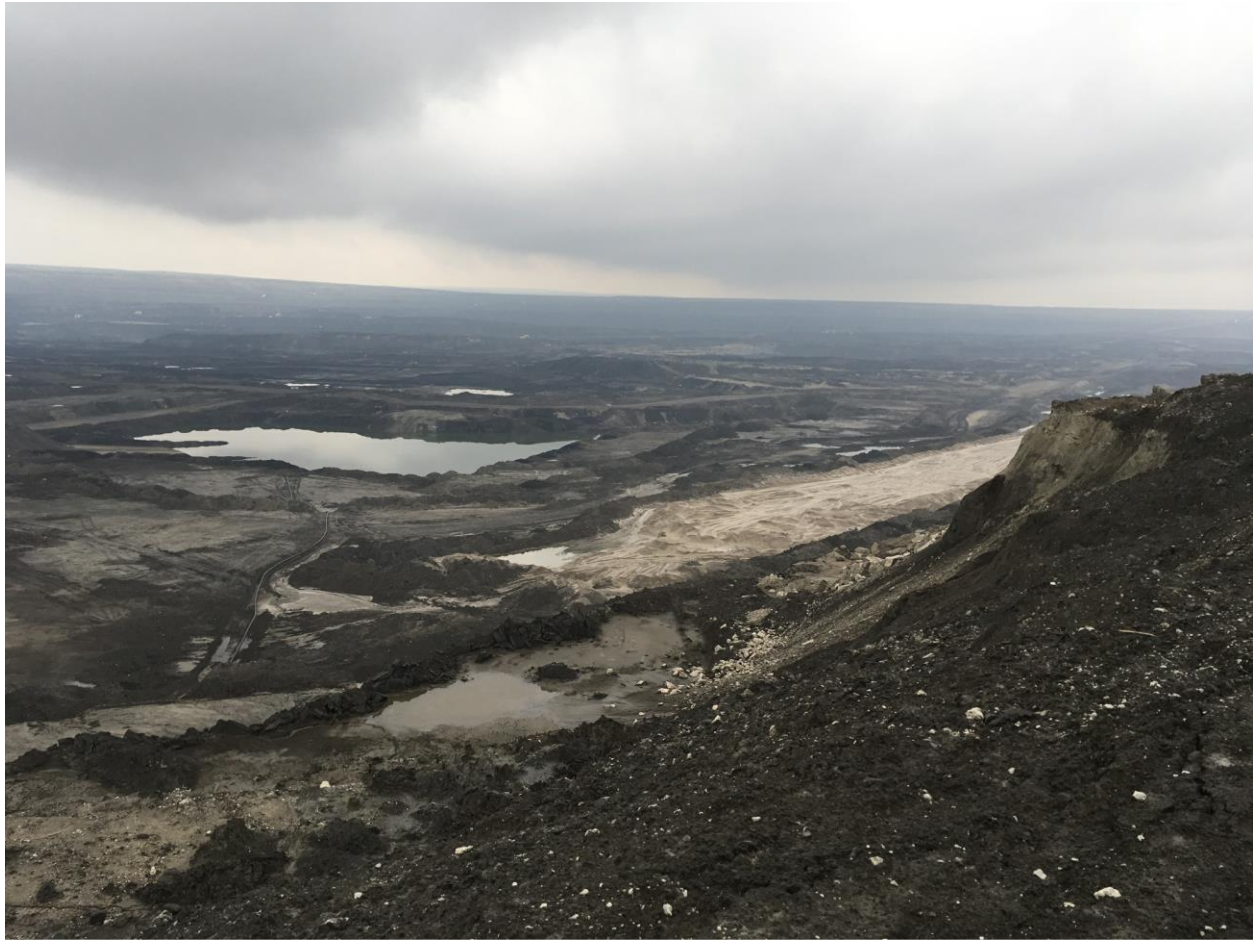
Summer Photo (b), Table 7. View of the open pit in winter conditions. Soft ground and standing water can be seen on bench.
