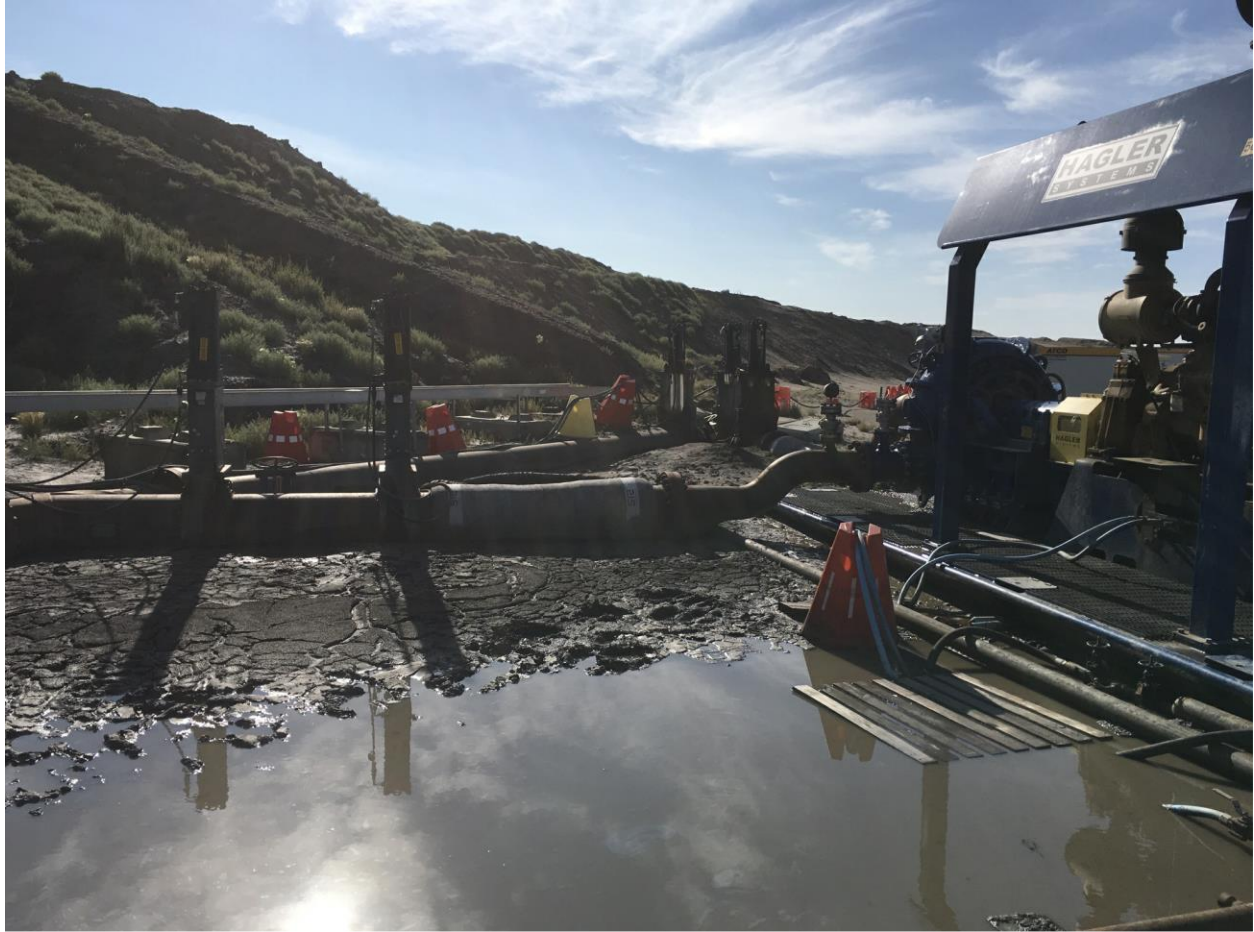
Summer Photo (g), Table 7. Pumps downslope of tailings pond dam. Pipes and associated structures in wet, soft ground conditions and adjacent to slopes.
