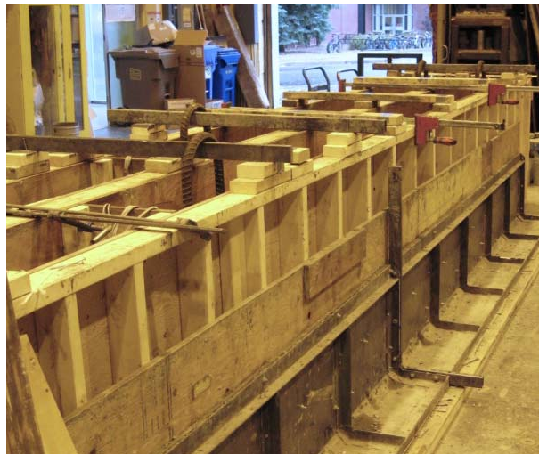
Figure 3-5: Formwork for h = 1000 mm specimens.
