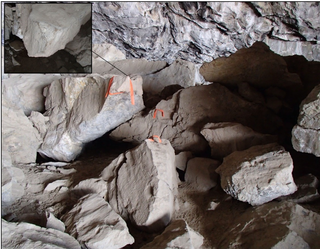
Plate 5.3. Smooth spots SS2, SS3, and SS4 in central rockfall area, with close up of SS2.
