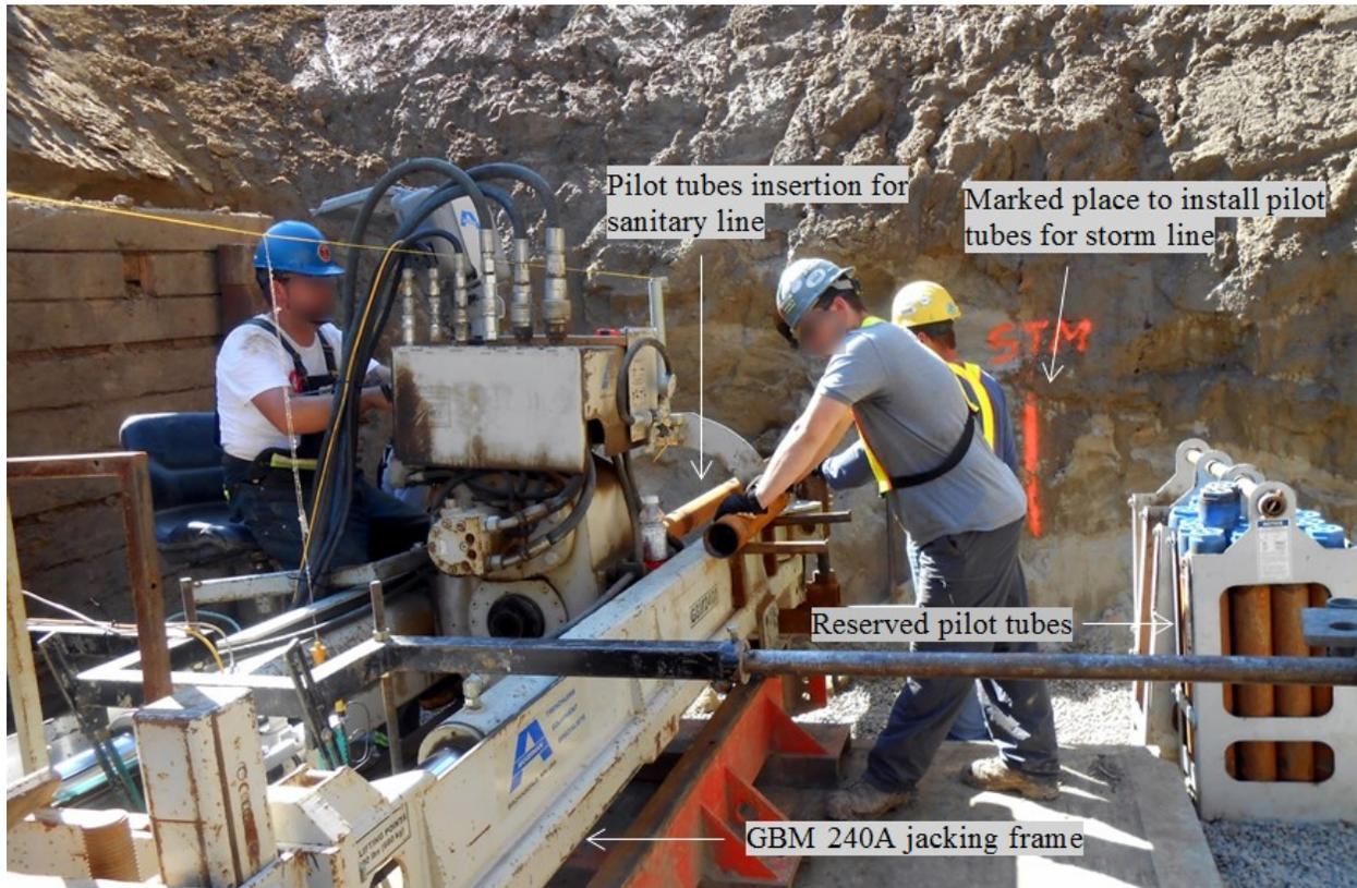
**Figure 3.2 Pilot tubes installation for sanitary line**
