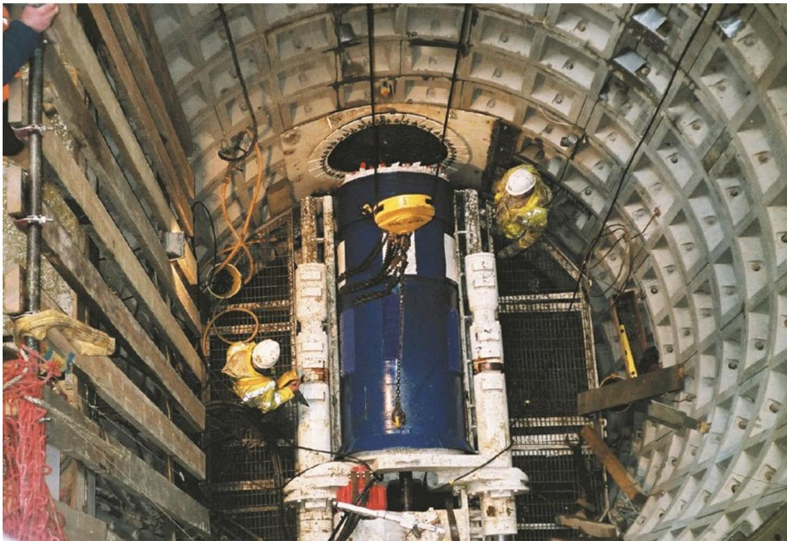
**Figure 2.12 Thrust shaft for pipe jacking process (PJA 2014)**
