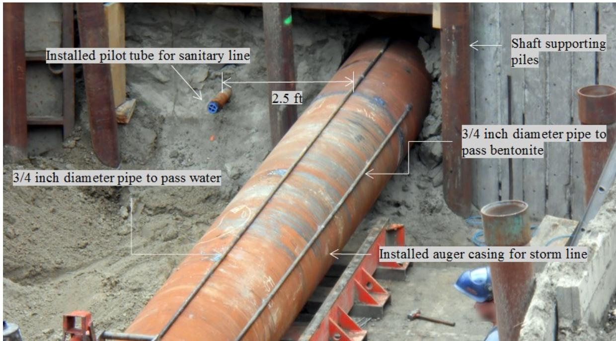
**Figure 3.3 Auger casing installation for storm line**
