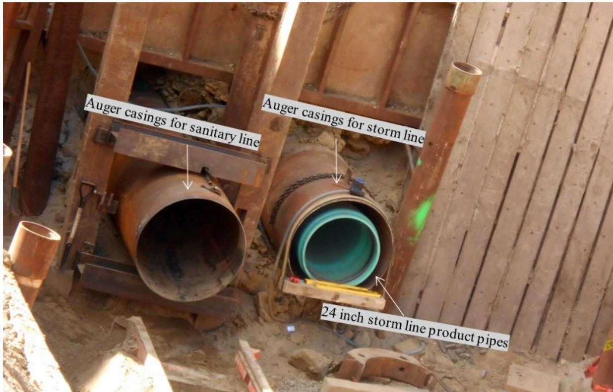
**Figure 3.5 Product pipes installation**
