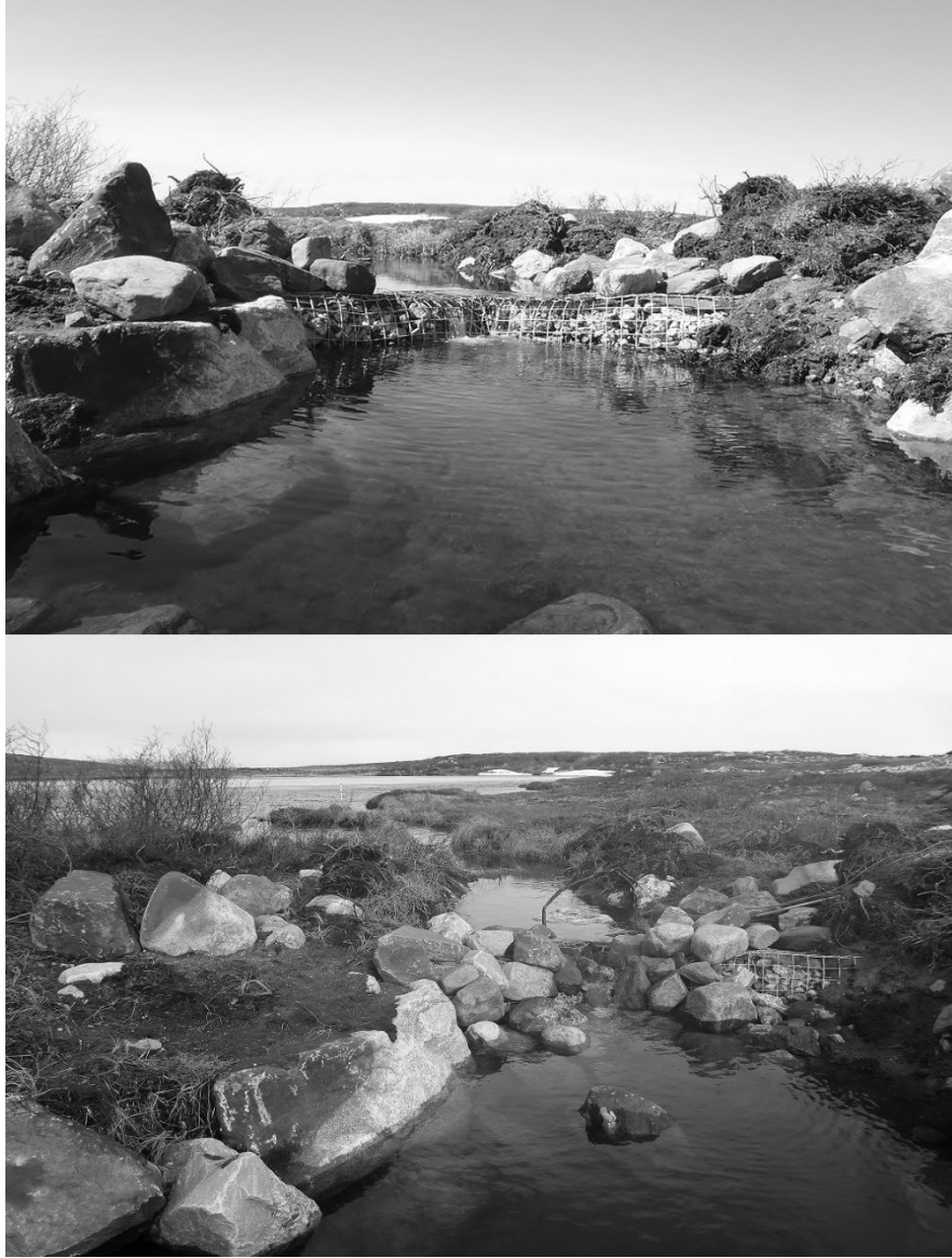
FIGURE 2.4.—A. M3S weir one (of six), facing upstream, 2 June 2012. This structure featured a 20 cm drop height and shallow ( < 3 cm) diffuse flows during the spring freshet, similar to other gabion-weirs during 2012. B. The same M3S structure, 5 June 2013. All gabion weirs were retrofitted for 2013 by notching their center to reduce sudden drops over weir structures, and to increase flow depths during low flows. The black hoop is the upstream PIT antenna. Photos by Fred Noddin
