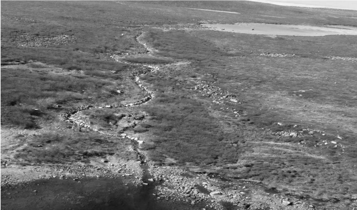
FIGURE 4.1.—The West Island nature-like fishpass during summer 2014. The lake in the upper-right portion of the photograph is West Island Lake, while the lake at the bottom of the image is Lac de Gras. This fishpass is approximately 300 m in length, and took five weeks to construct during autumn 2012. Photo by Fred Noddin.
