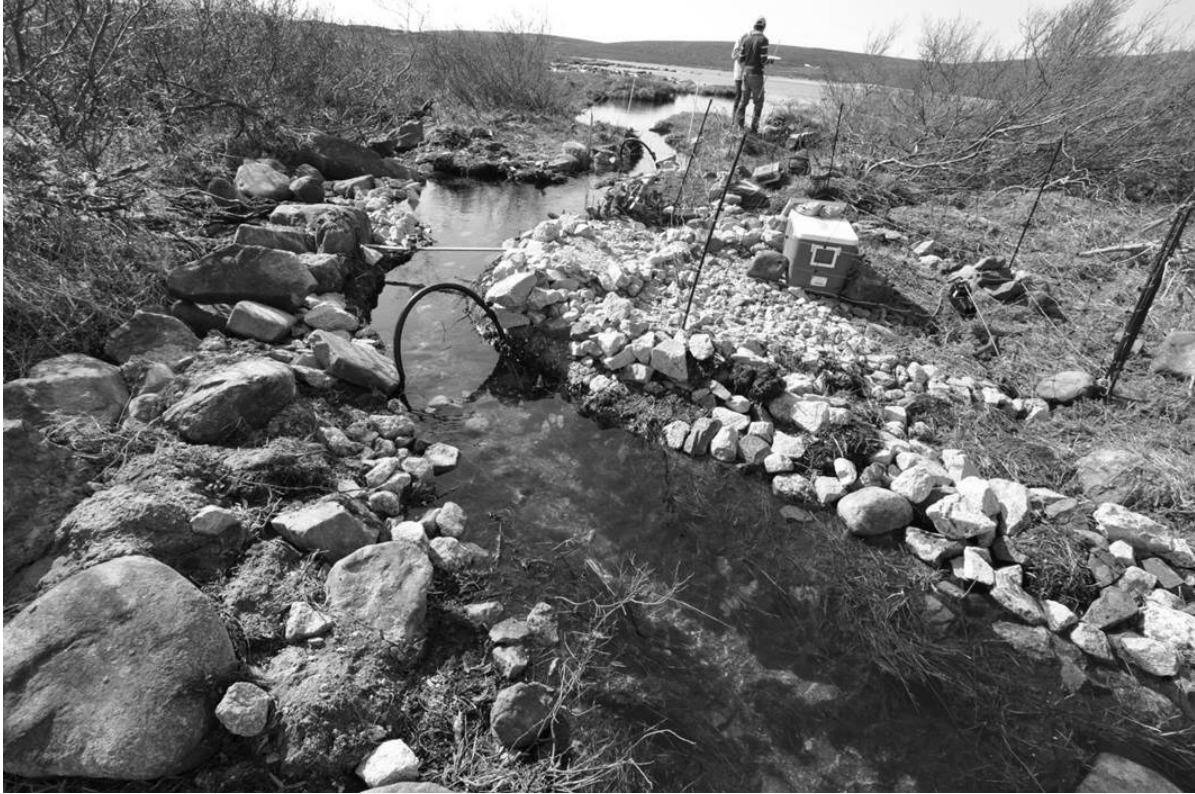
FIGURE 2.3.—Nature-like choke-pool fishpass (M2S), facing downstream, 4 June 2013. The black hoop is the upstream PIT antenna, the constricting “choke” is immediately behind this antennae, and the relatively wide “pool” is immediately downstream of the choke. This fishpass was not retrofitted for 2013. Photo by Fred Noddin.
