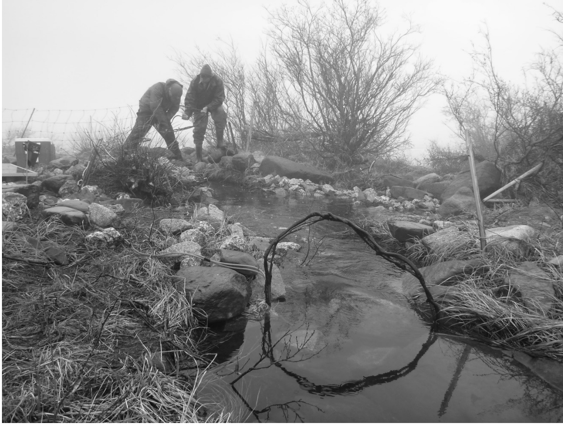
FIGURE 2.3.—Nature-like choke-pool fishpass (M2S), facing downstream, 4 June 2013. The black hoop is the upstream PIT antenna, the constricting “choke” is immediately behind this antennae, and the relatively wide “pool” is immediately downstream of the choke. This fishpass was not retrofitted for 2013. Photo by Fred Noddin.
