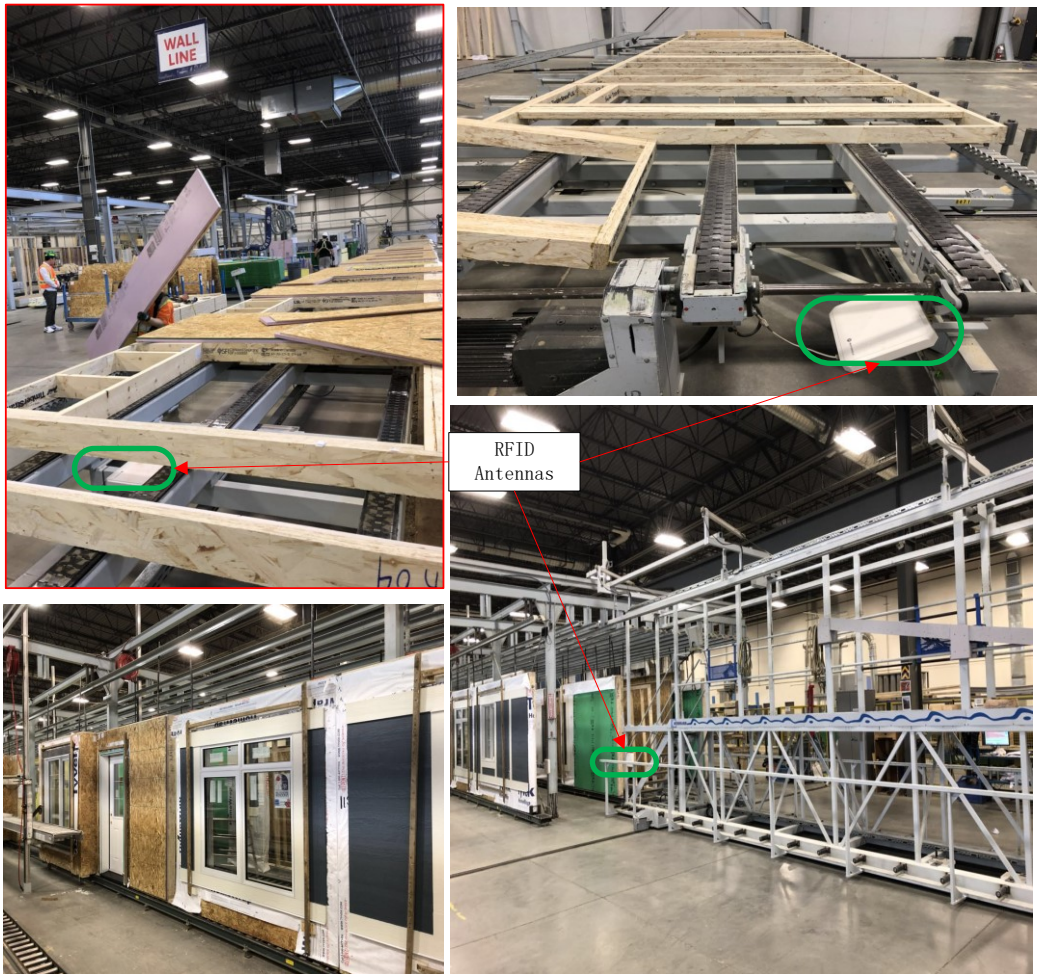
Figure 5-1. RFID System on Wall Production Line (Courtesy of ACQBUILT, Inc.)
