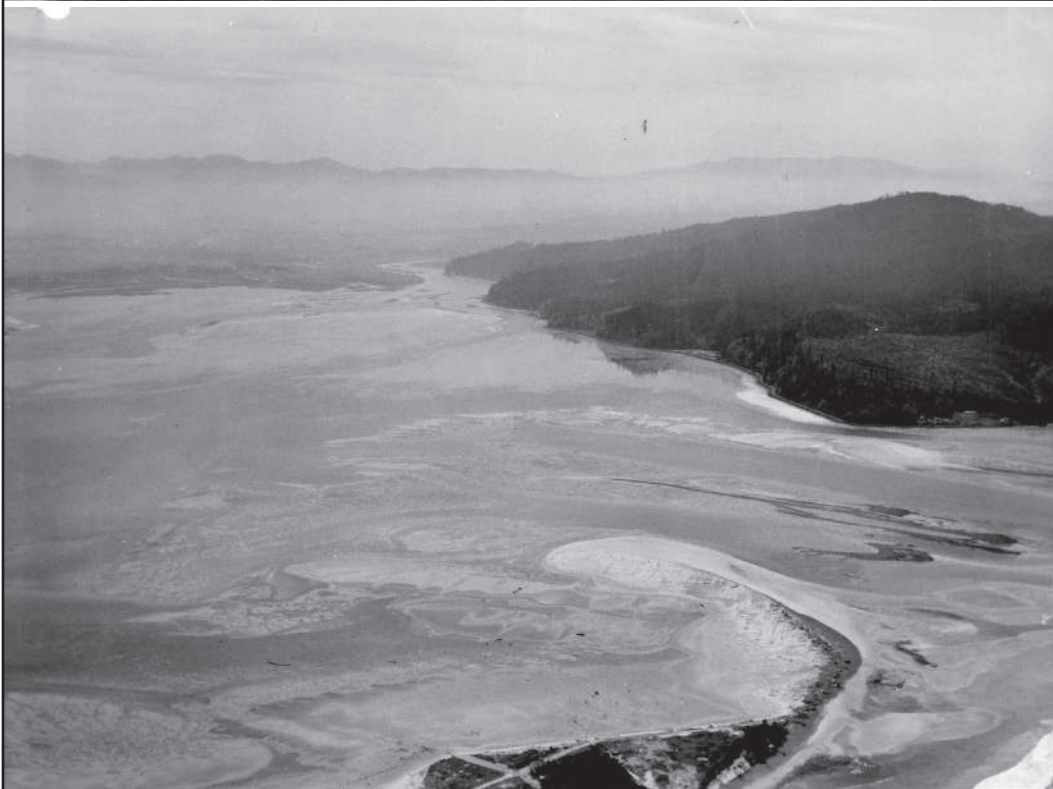
Figure 1-4. Historical photographs of the Bayocean Peninsula storm breach (View #2). Both photos: aerial views to the southeast. Tillamook River mouth can be seen in the background. Note presence of the sand ridge curving into the bay, and attached to the main part of the spit. Photos courtesy of Tillamook County Pioneer Museum, used by permission.
