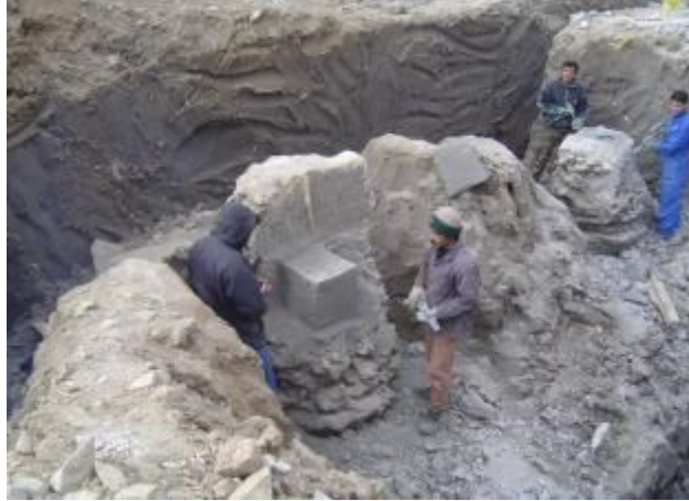
Figure 3-64 Soilcrete columns and block samples (B Nikbakhtan and Osanloo 2009)
