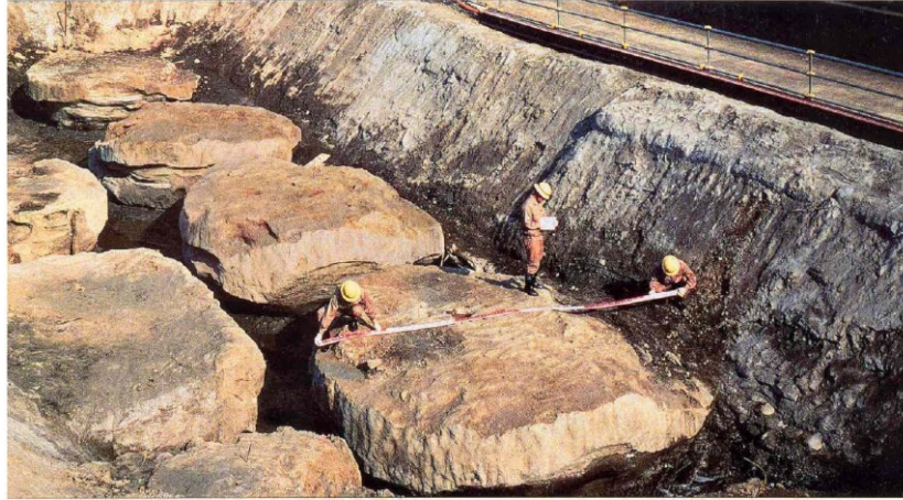
Figure 3-15 Soilcrete columns in sandy soil formed by super jet grouting (Superjet 2004)
