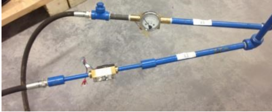
Figure 4-18 Flow meters in grout and water line
