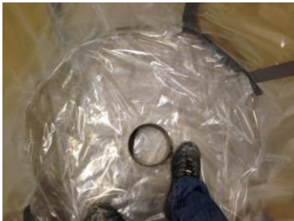
Figure 6-5 Jet grouting tank wrapped with thick plastic
