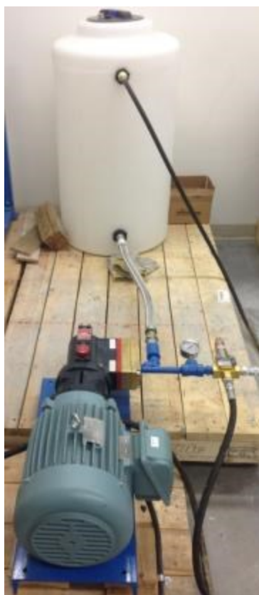
Figure 4-15 Water jetting plant
