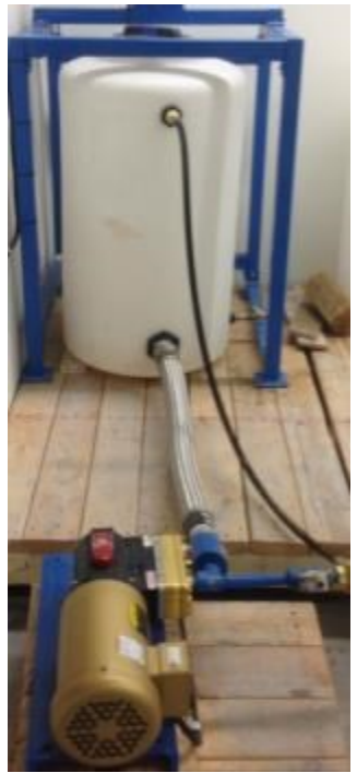
Figure 4-17 Grout jetting and mixing plant
