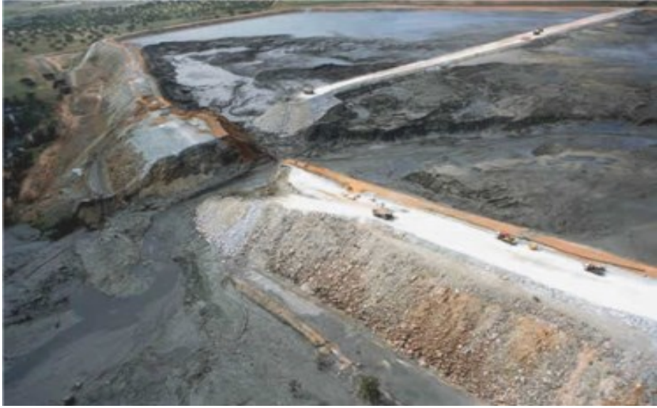
Figure 7-1 Los Frailes tailing dam failure (Mech 2011)
