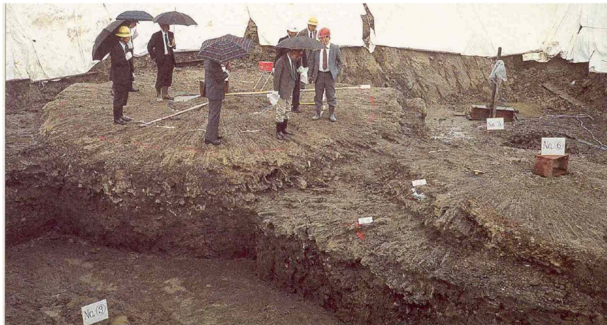
Figure 3-14 Soilcrete columns in clayey soil formed by super jet grouting (Superjet 2004)
