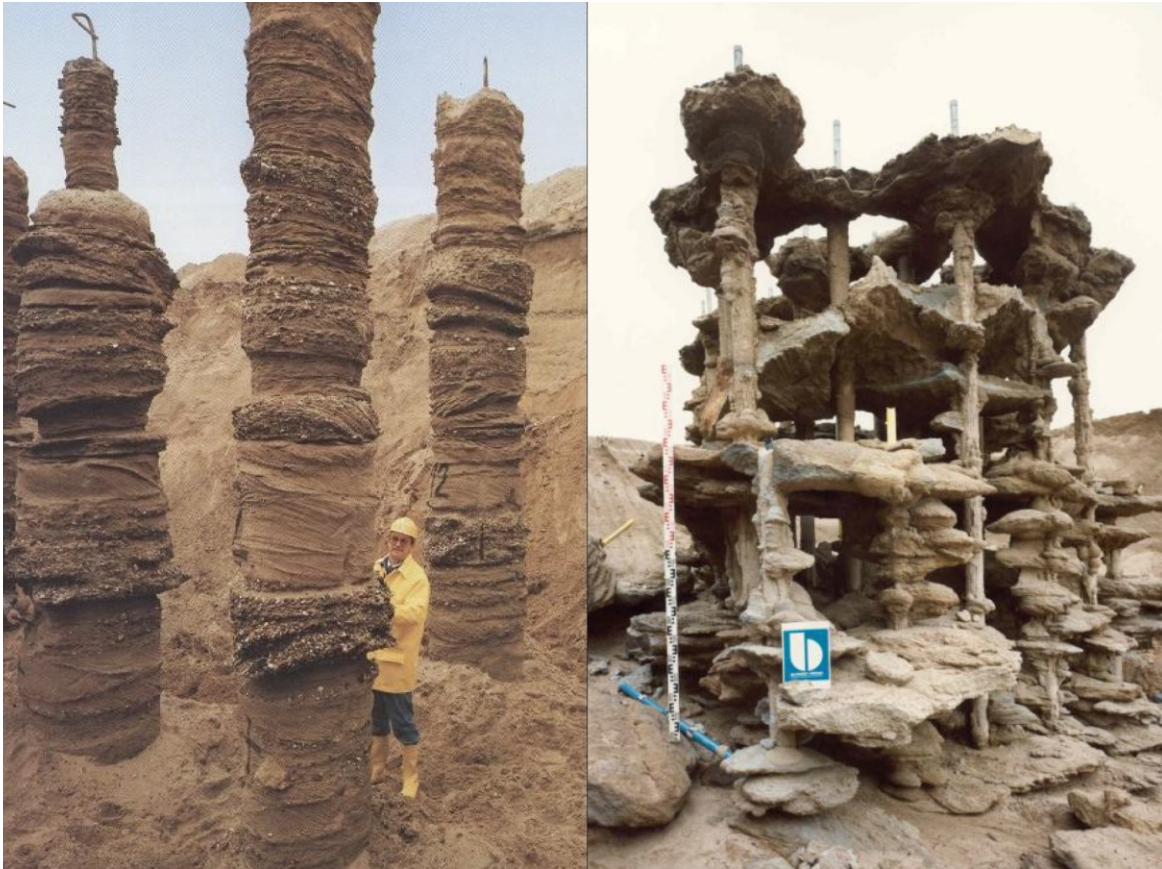
Figure 3-4 Jet grouting (left) v.s. low pressure conventional grouting (right) (Foundations 2012)
