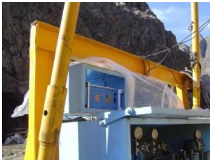
Figure 4-6 Control panel of jet grouting operational parameters
