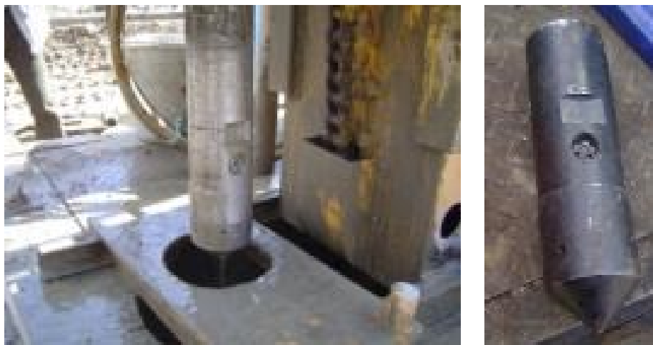
Figure 4-9 Triple fluid jet grouting monitor
