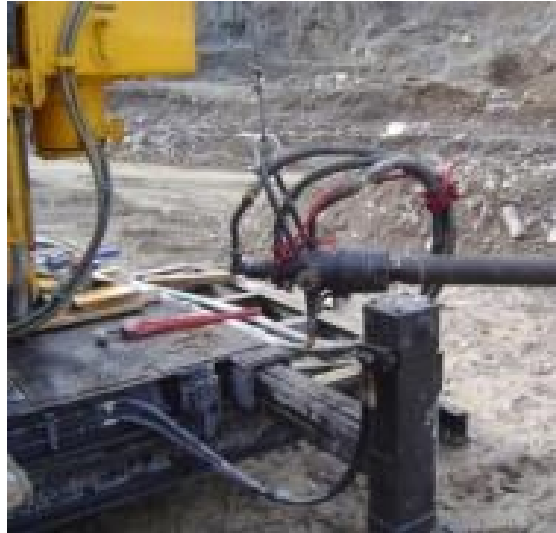
Figure 4-7 Water, grout and air swivel jointed to the rod
