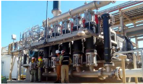
Figure 4. A 1.000 m 3 /hr Piston diaphragm pump
