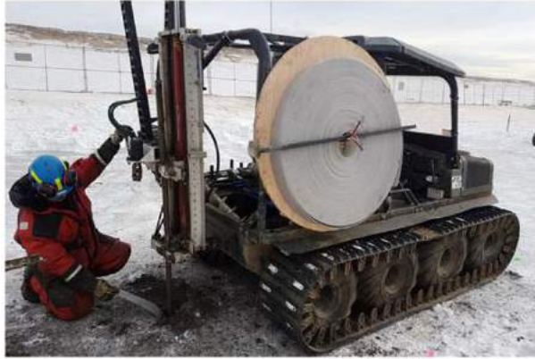
Figure 2. Argo-mounted wick drain deployment system
