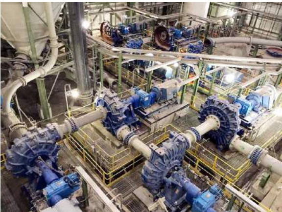
Figure 3. Centrifugal pumps in series
