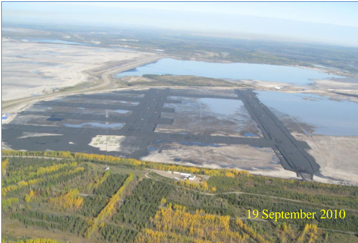
Figure 3-14 Constructing Coke Cap Over Suncor Pond 5
