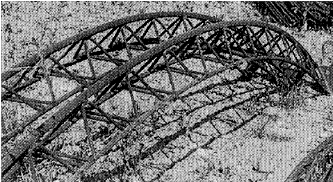
Figure 4.14 - Lattice girders prior to installation
