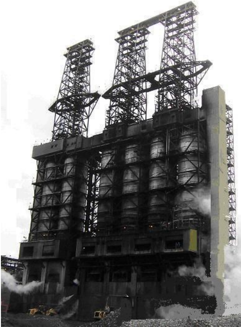
Figure 1.5 – Coke Drum Unit Derrick Structures
