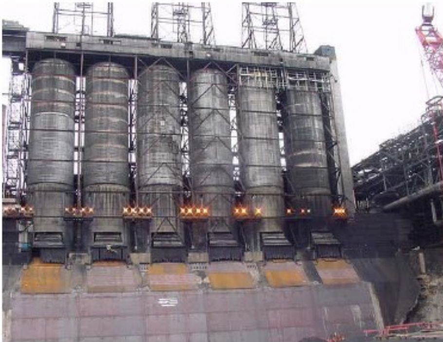
Figure 1.1 Photograph of Coke Drums in a Process Unit
