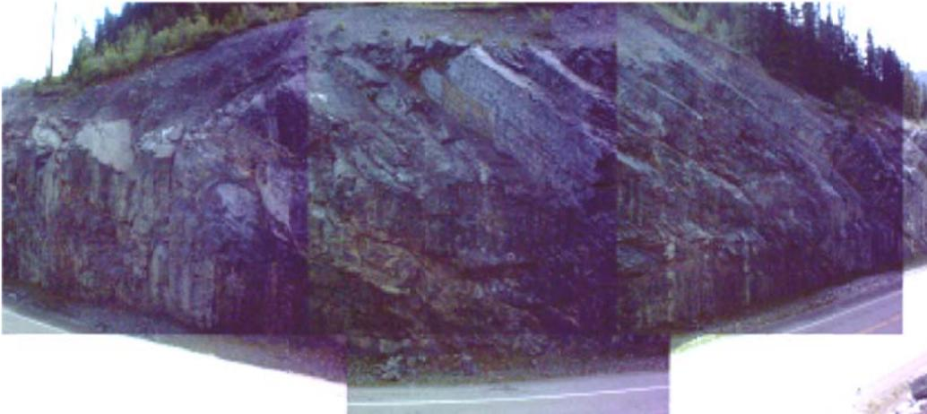
**Figure 3.15: Composite Image of Galatea Creek Through-Cut Stitched Together from ILRIS-3D Camera Images**
