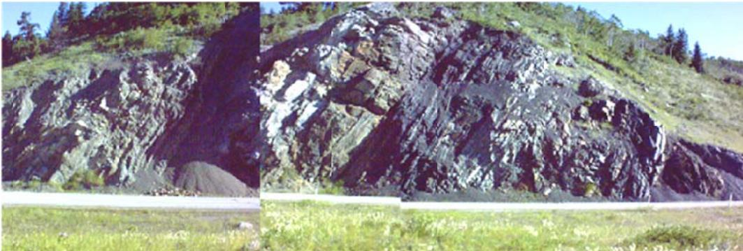
Figure 3.13: Fir Creek Rock-Cut as Stitched Together from ILRIS-3D Camera Images
