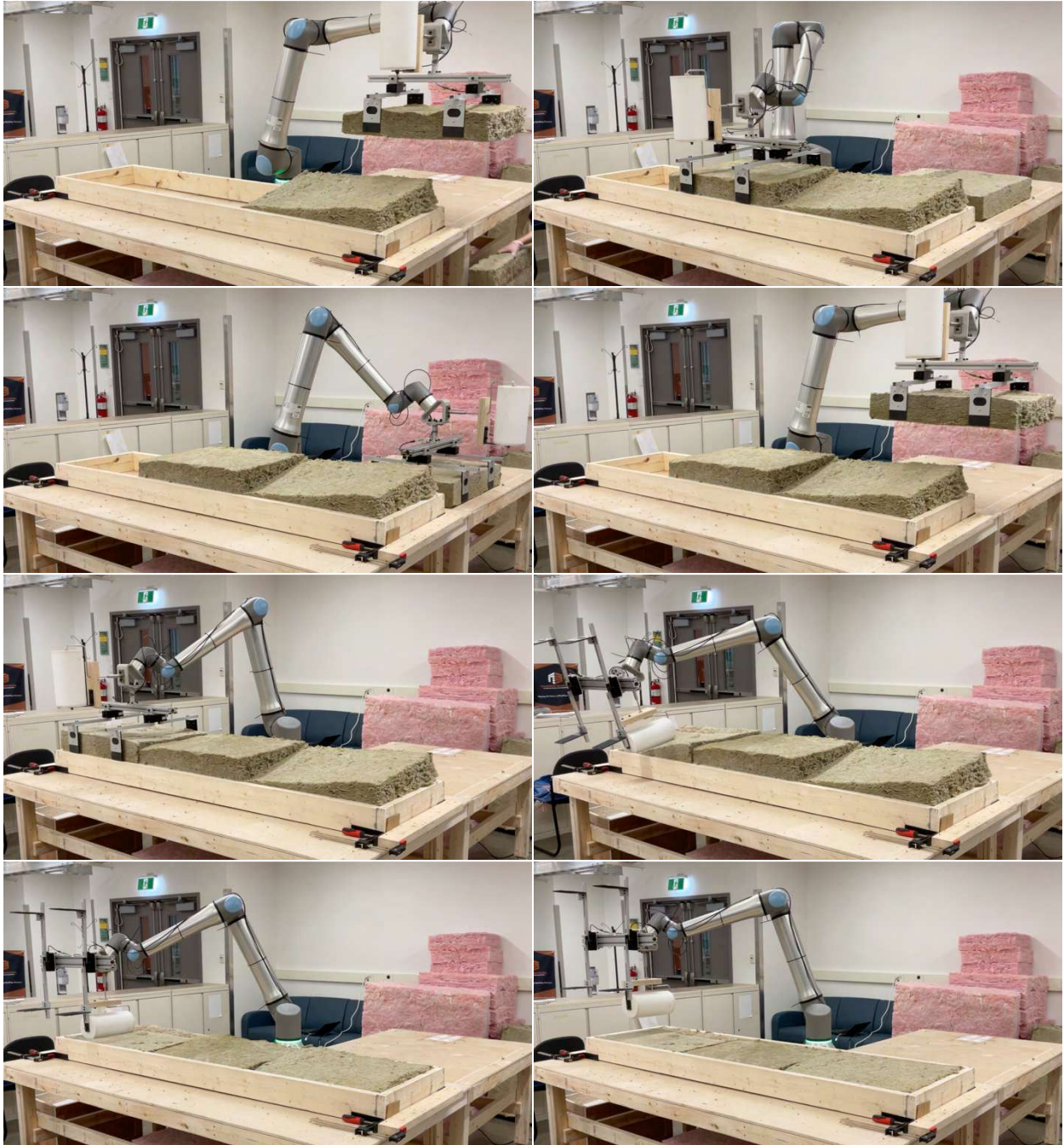
Figure D.21: H-GLPPR process for Scenario 3 with 23 x 5.5-inch (584 x 140 mm) fiberglass insulation
