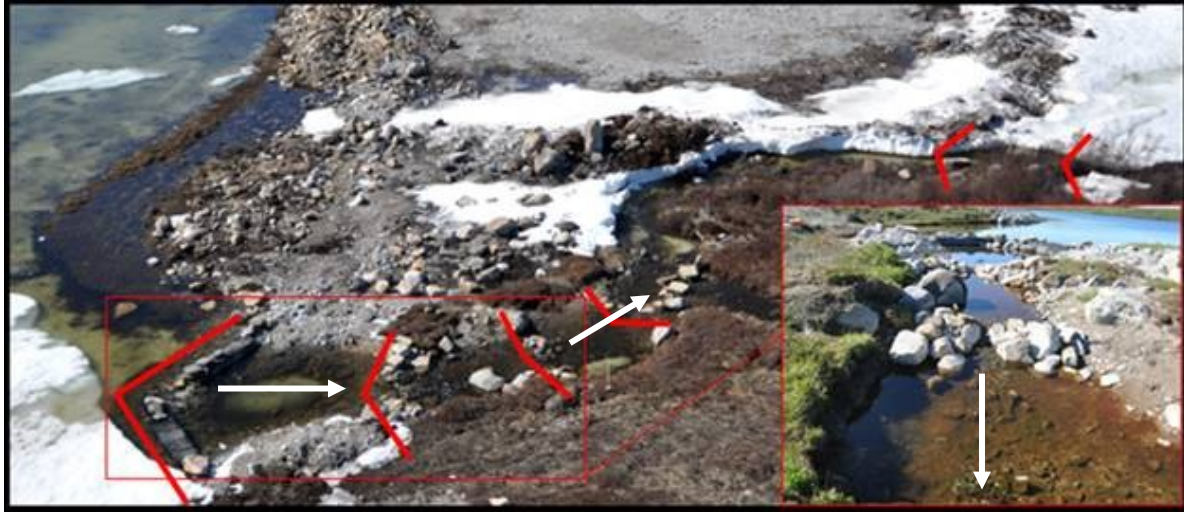
Figure 1-6. Gabion-weir treatment at M1S. M1L (upstream) is to the left. Red bars indicate gabion weir locations, white arrows indicate direction of flow, and red box indicates location of photo insert (looking upstream to M1L) depicting more detail of step-pool structures after retrofitting in fall, 2012. Photo taken June 2, 2013, insert photo taken June 27, 2013.
