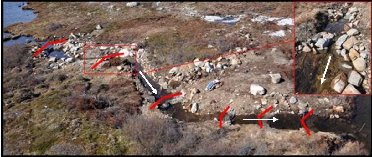
Figure 1-8. Gabion-weir treatment at M3S. M3L (upstream) is at the upper left; M1L (downstream) is at the lower bottom. Red bars indicate gabion weir locations, white arrows indicate direction of flow, and red box indicates location of photo insert depicting more detail of step-pool structures after retrofitting in fall, 2012. Photo taken June 12, 2012, insert photo taken June 9, 2013.
