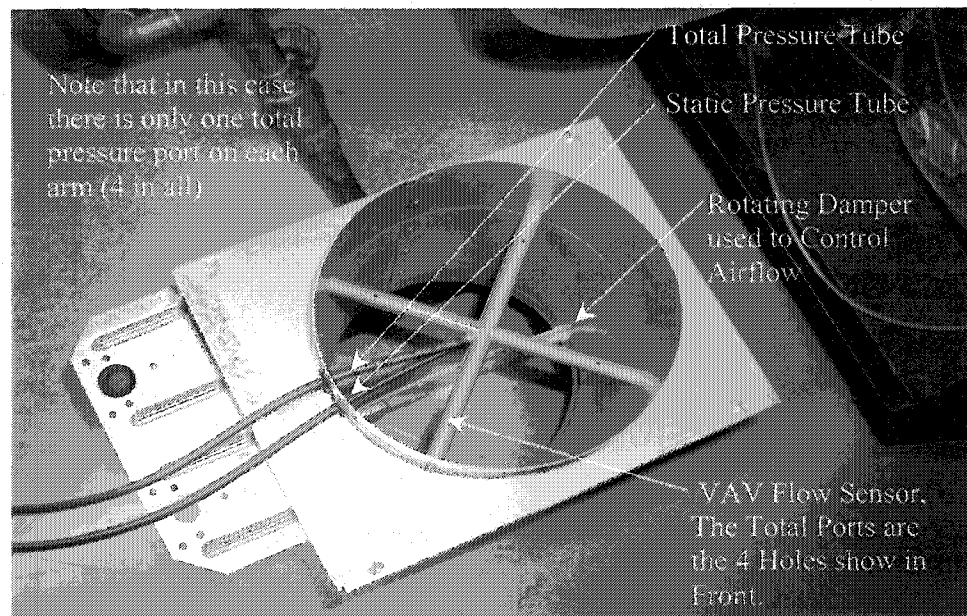
Figure 2: Internals of a typical VAV terminal where the flow sensor (blue) is located prior to a circular damper. The total ( P_T ) and static ( P_S ) pressure signals are recorded through the red and green tubes that stretch between the center of the flow sensor and the outside of the duct. The following fluid mechanics analysis indicated that if the total pressure ( P_T ) were recorded along the outside of the duct (i.e. the red tube circled the duct and the arms attached to it from outside the duct) then this would minimize a possible error term. Unfortunately, the current configuration is quite common due to its easy assembly and inexpensive manner.
