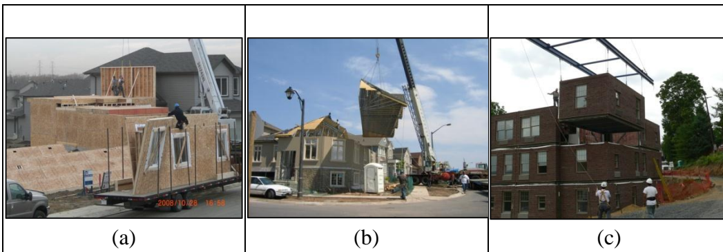
Figure 3-1: On-site installation of prefabricated building components
