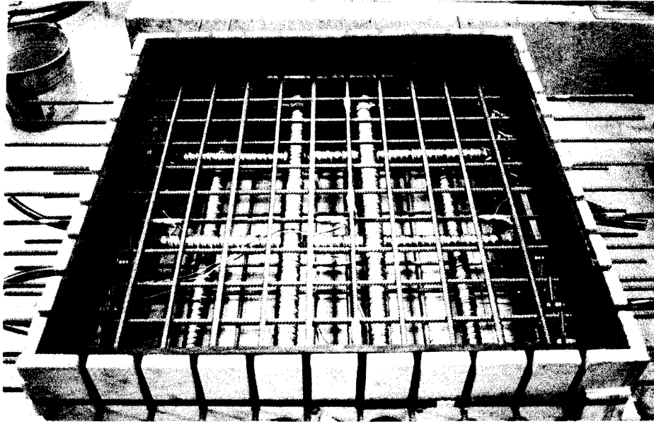
Figure 2.7 Segment 10 Prior to Casting
