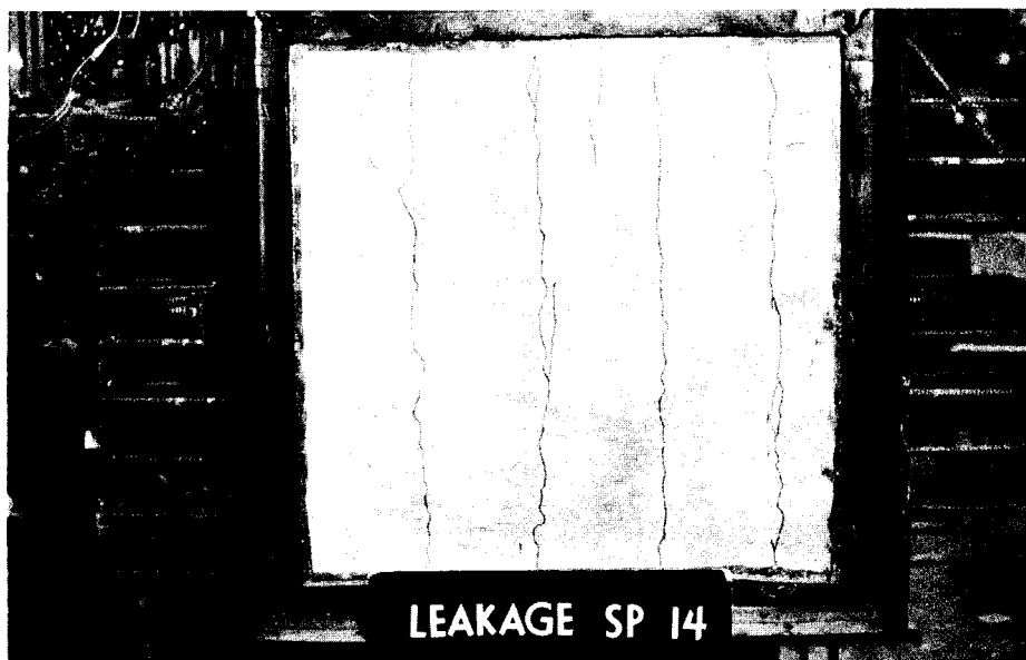
Fig. 5.11 Down-Stream Face of Segment 14 After Testing
