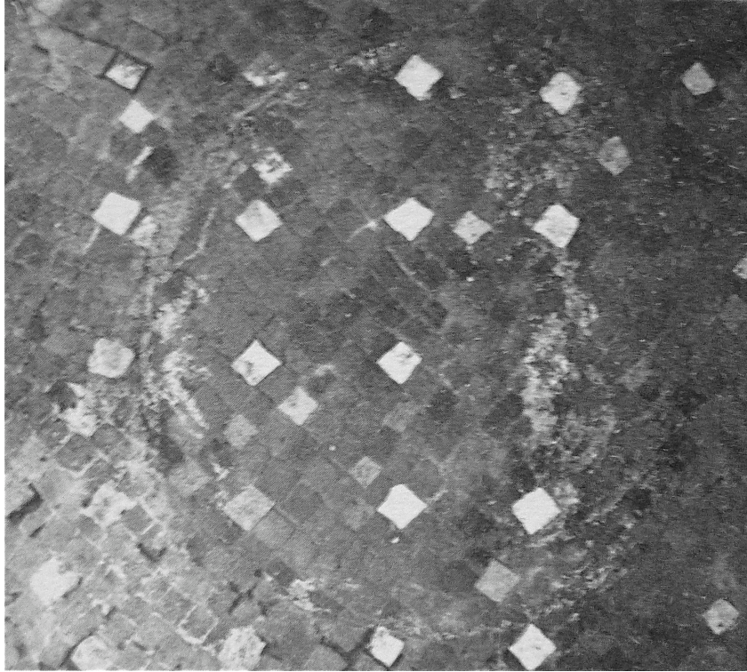
Figure 3.19 Photograph, Discolouration on mosaic in Room A8, Villa Prato, Sperlonga from X. Lafon (1991) "Les bains privés dans l'italie romaine." Figure 8, p. 105.
