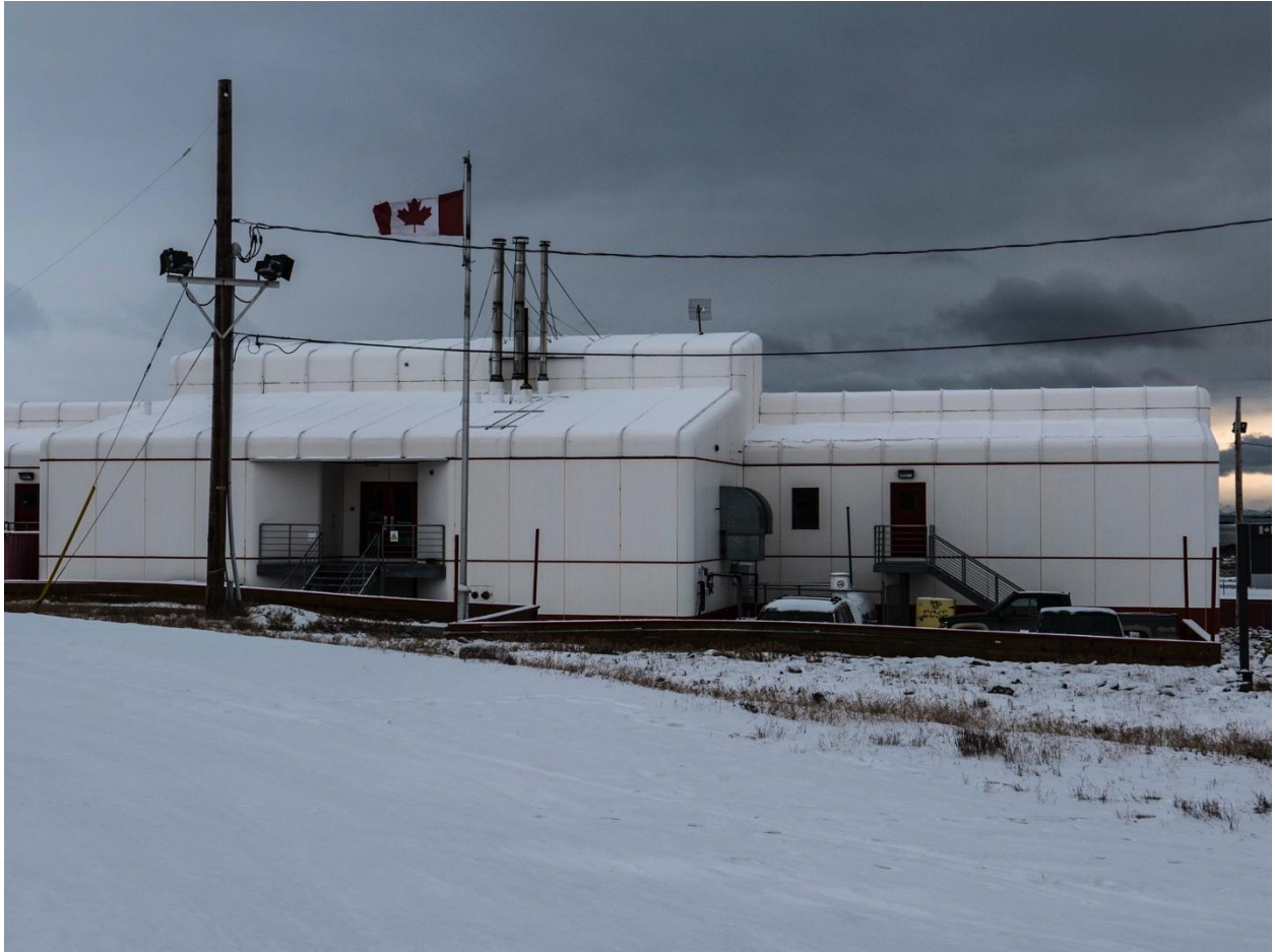
Plate 1.4 Pre-fabricated buildings in Iqaluit.
