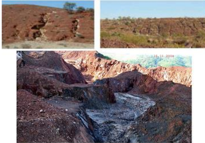
Figure 4: Gulling failures in dumps (Sankar, n.d.)
