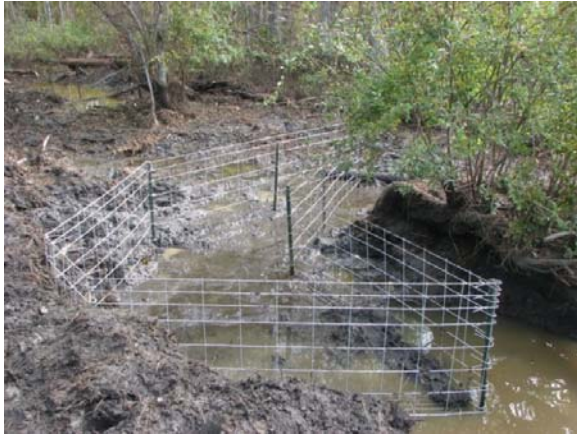
Plate 1. Beaver management device installed at culvert location was used as an example of human-nature partnership in conservation.
