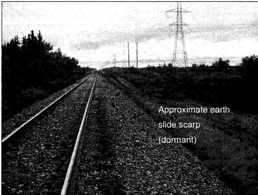
Figure 8-10 Case example of an Earth (Embankment) Slide – Compression hazard scenario at Mile 122.7 of CN Vegreville Subdivision (photos by Tim Keegan, CN file 4670-VGR-122.7)
