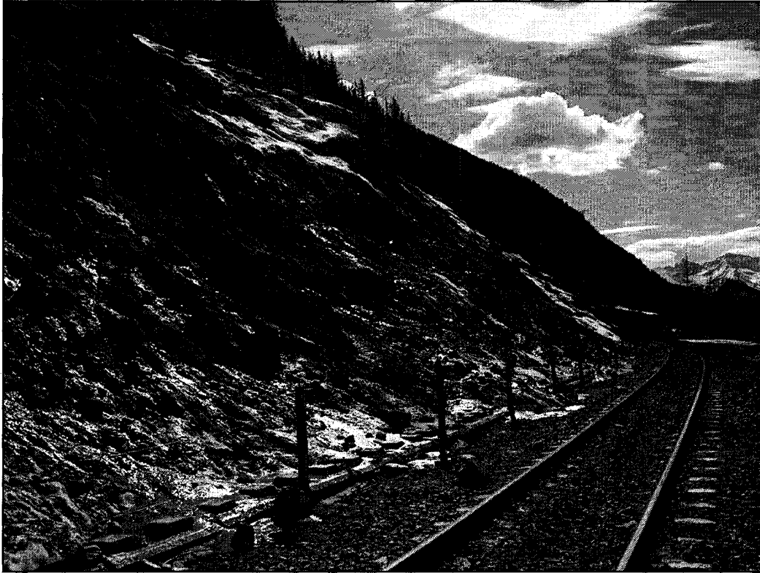
Figure 7-9 Example of ground frost, a preparatory causal factor, melting and triggering debris falls at Albreda Subdivision Mile 54.55 (Photo by Tim Keegan taken April 4, 2006).
