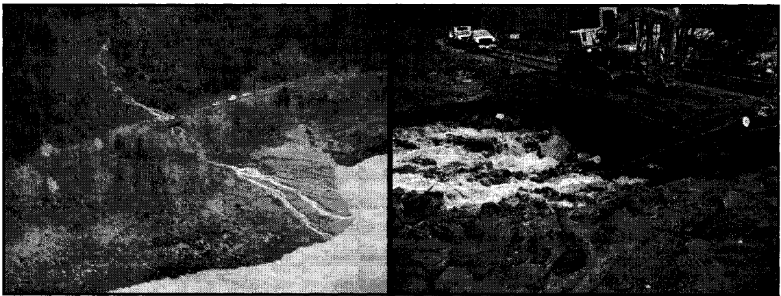
Figure 11-23 Case example of a Channel Aggradation / Debris Flow - Avulsion - Local Scour / Seepage Erosion / Gully Erosion hazard scenario involving a debris flow and track failure by blockage at Mile 20.3, CN Yale Subdivision (photos by Tim Keegan Nov 16, 2007, CN file 4670-YLE-20.3)
