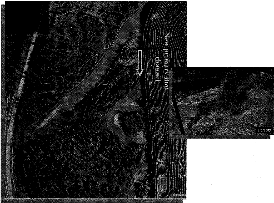
Figure 11-16 Case example of an Avulsion - Bank Erosion / Local Scour / General Scour - Earth Slide hazard scenario at Mile 112.1 of CN's Albreda Subdivision (Aerial photo from Zorkin, (2005), photo by Tim Keegan)
