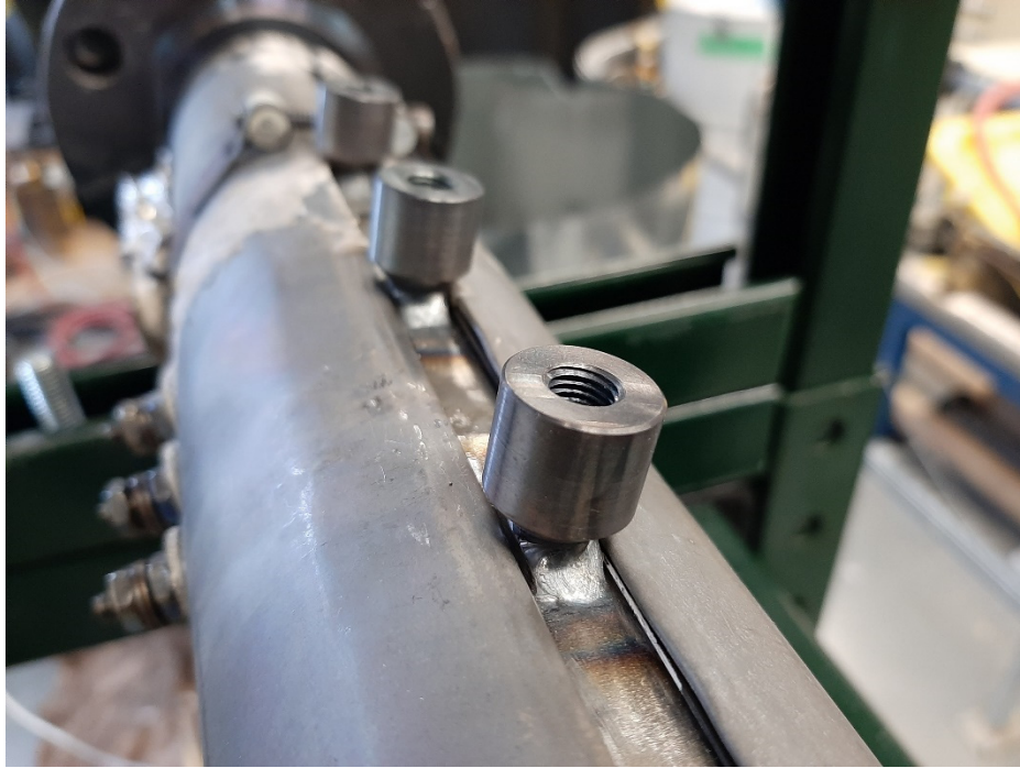
Figure 3.10 A photo of the threadolets welded on a pipe in the test section for connecting the pressure transducer ports to the pipe via straight male fittings.
