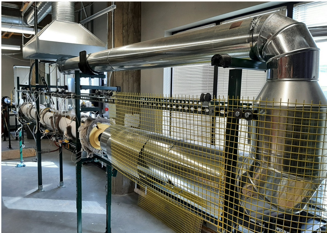
Figure 3.2 A photo of the pipe flow setup covered with insulation and a protective shield.
